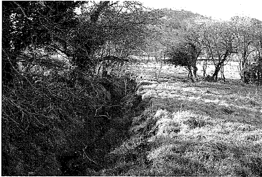
Plate 7- Open ditch with small flow open to field
