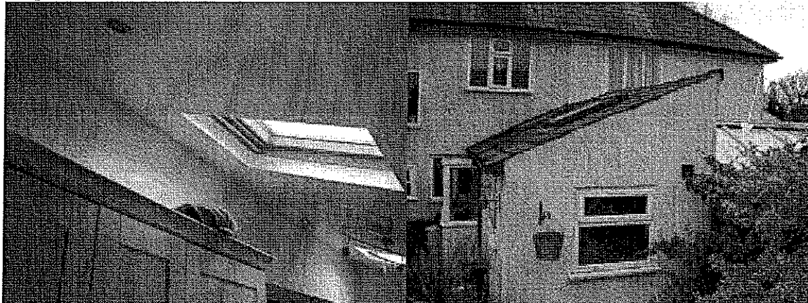
P3 Inside present extension - no void
