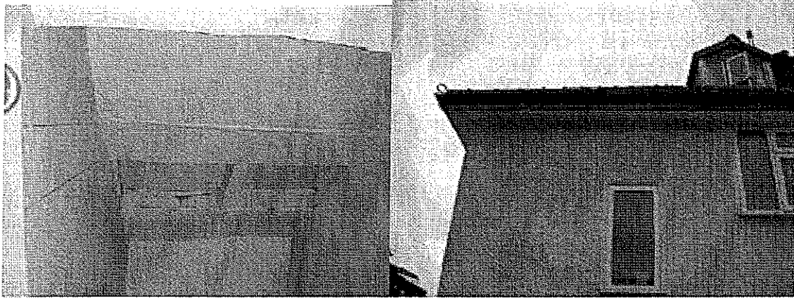
P1 part of boarded loft at eaves
