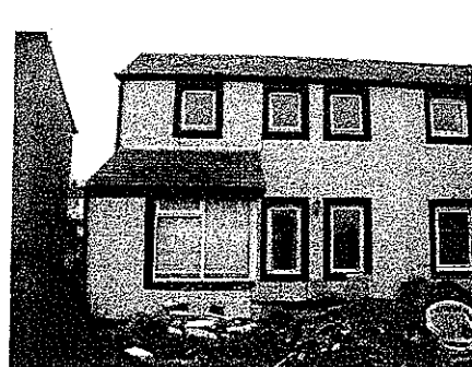
Figure 3: rear (west) elevation
