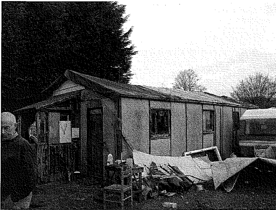
Demolition of former Women's Institute Building and Erection of Dwelling at land adjacent to Lynbrook, Longsight Road, Clayton le Dale, BB1 9EX
