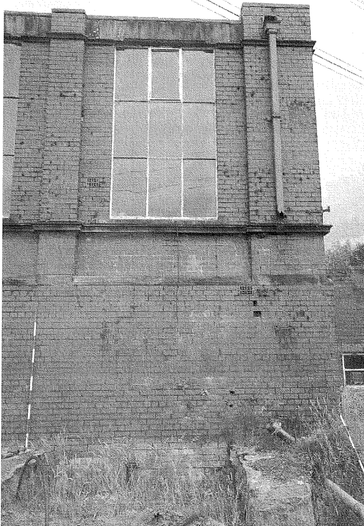
Plate 6 South Elevation window and brick detail
