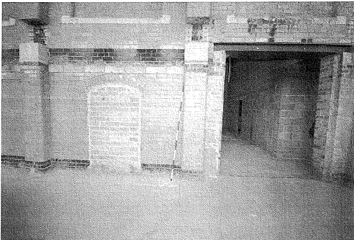
Plate 13 Blocked door and new opening
