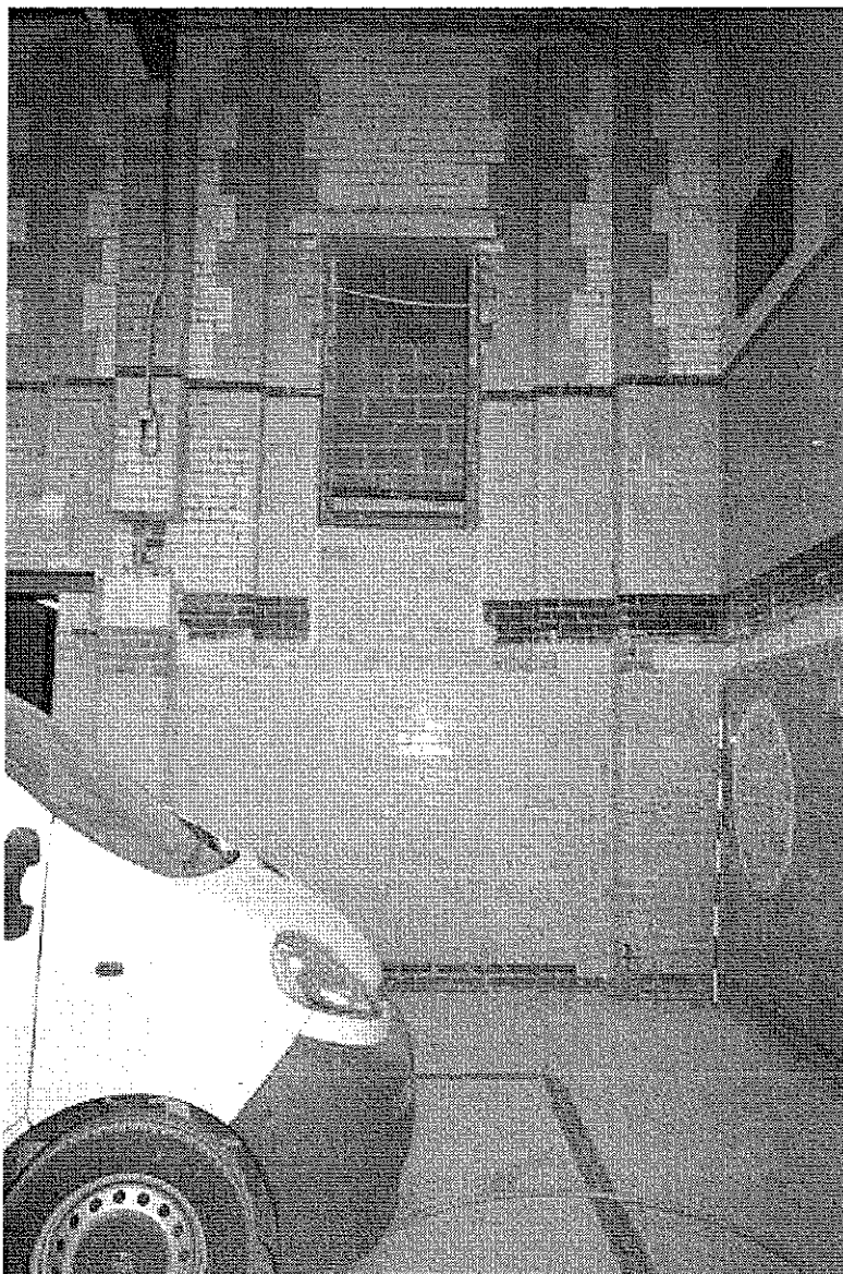
Plate 12 Showing where mezzanine floor has been removed
