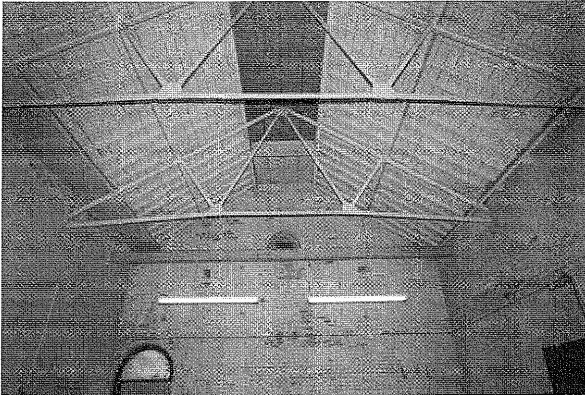
Plate 17 Roof Structure North-West
