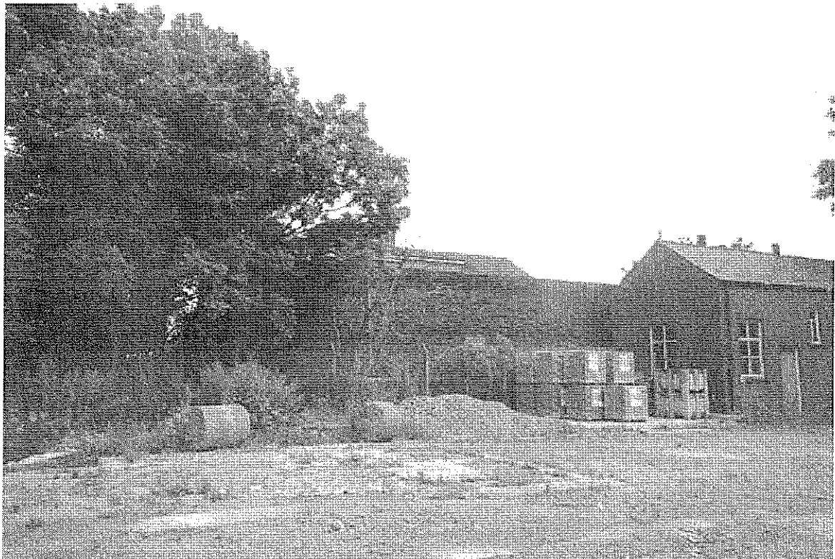
Plate 33 South Elevation Sub-station
