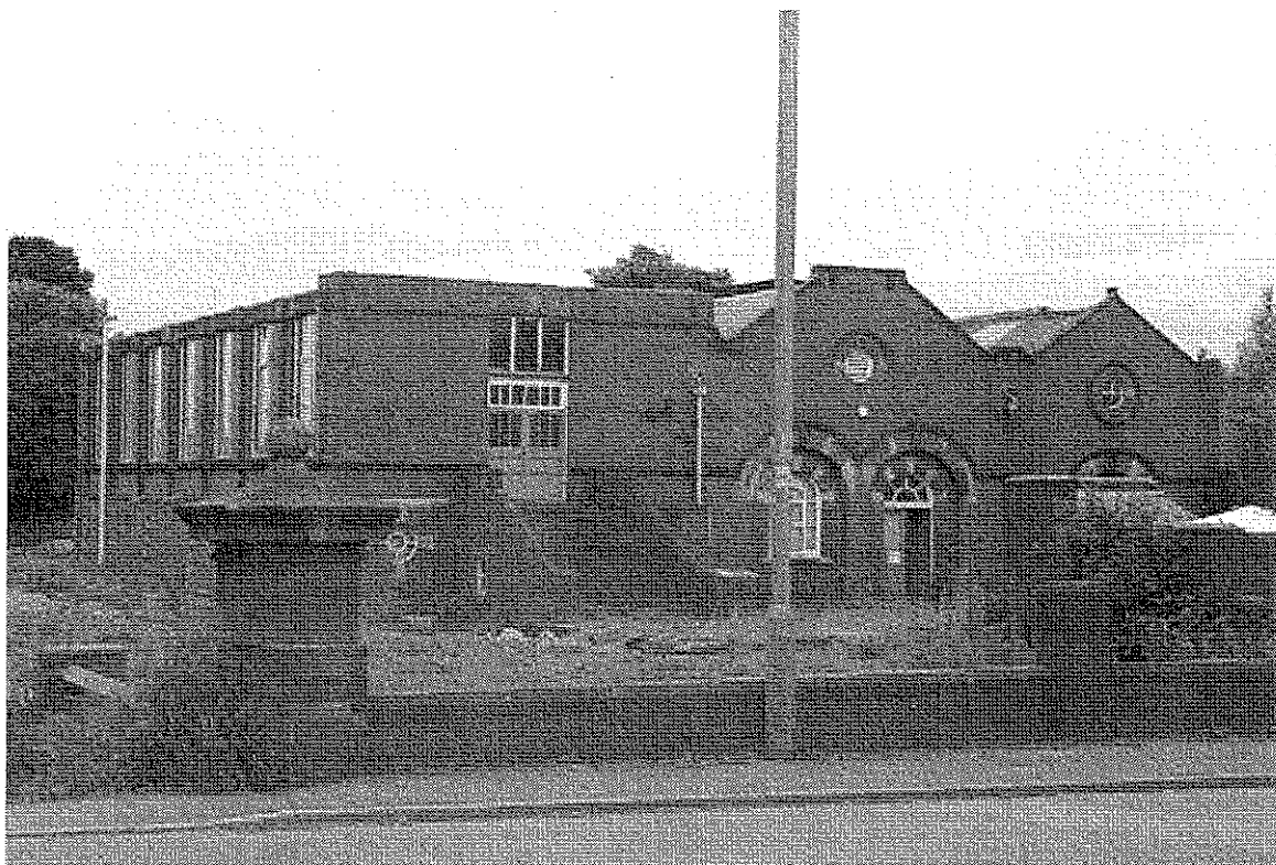
Plate 37 Boundary Wall with stone capped pier
