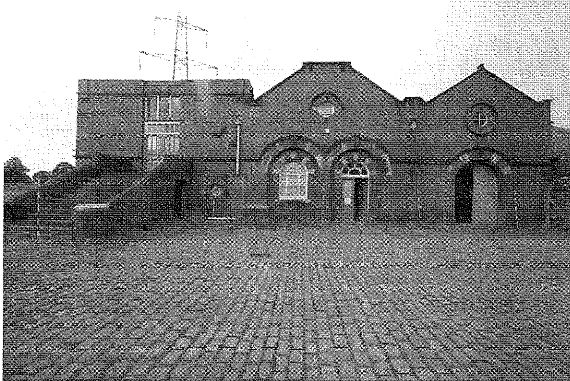
Plate 1 The Front (East Elevation)
