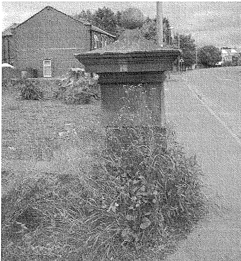
Plate 36 Stone Capped Wall Pier South-West corner of the land
