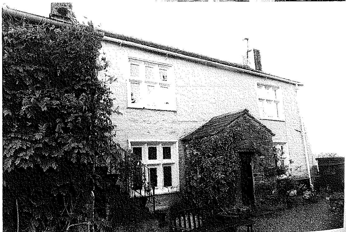
Photo 12 Frontage to Rodhill Gate Farm:
