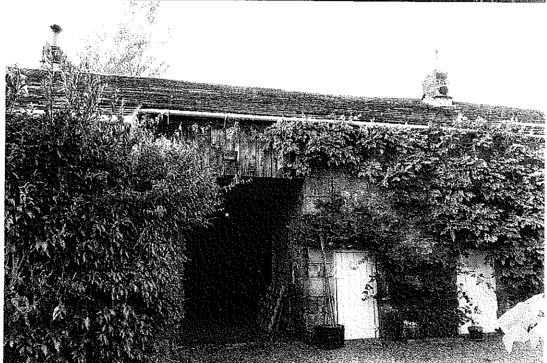
Photo 9 Abutment of Barn & part of Radhill Gate Farm
