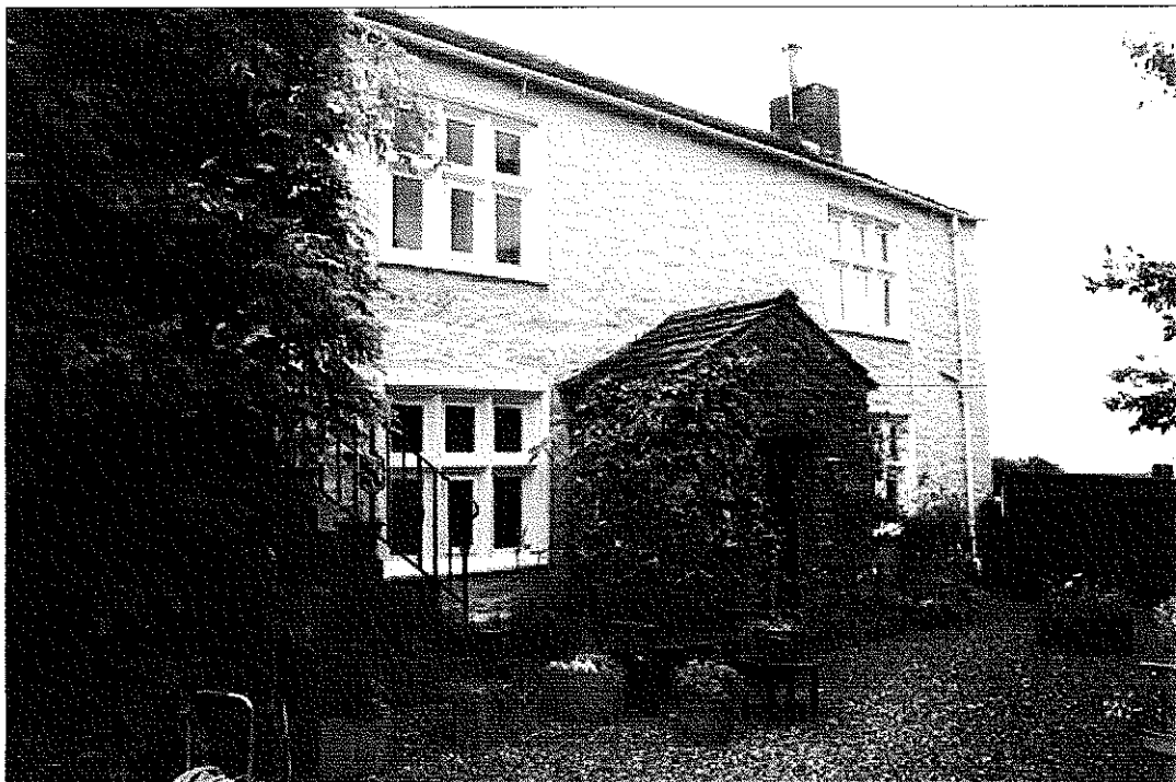
5 Rodhill Gate Farm from the south
