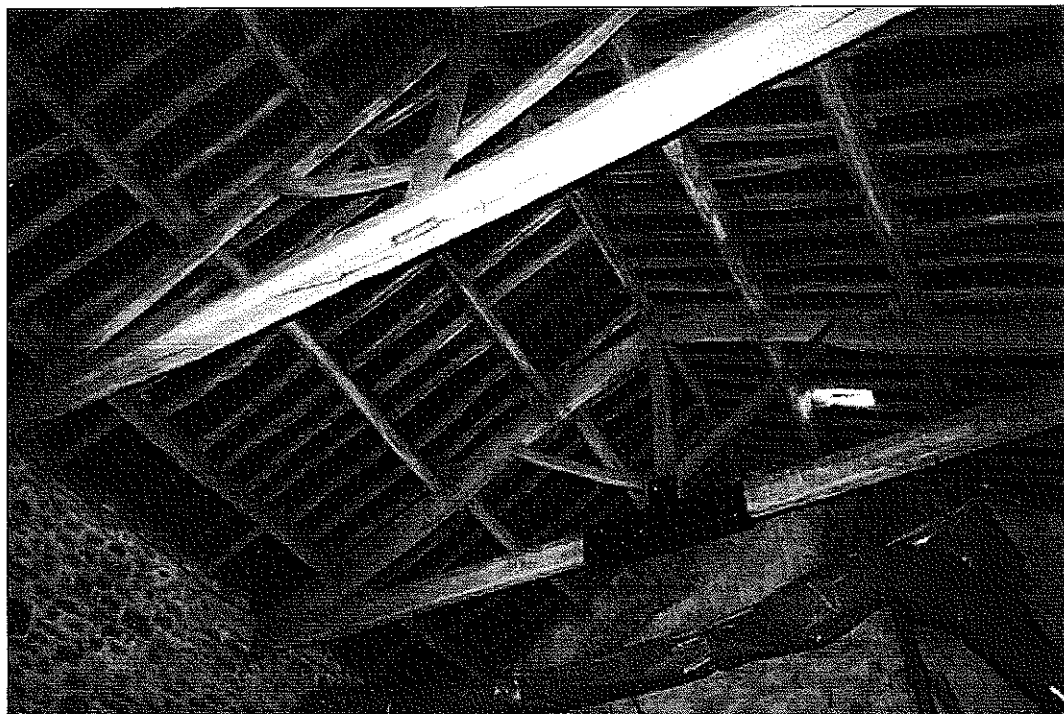
12. Kingpost roof trusses above the barn
