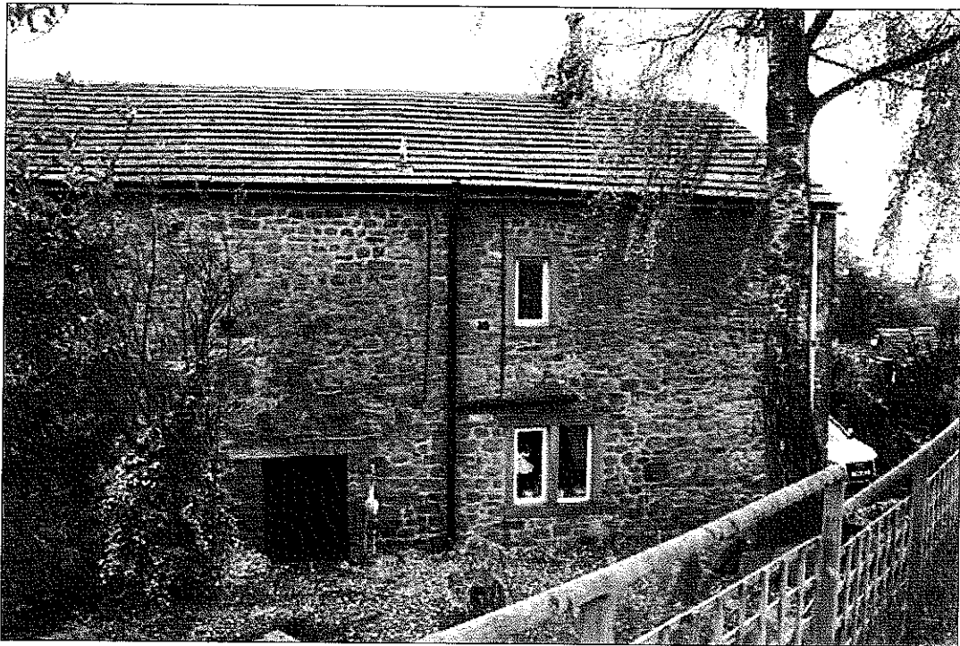
16 Northwest elevation of Rodhill Lodge (property begins right of door to barn)
