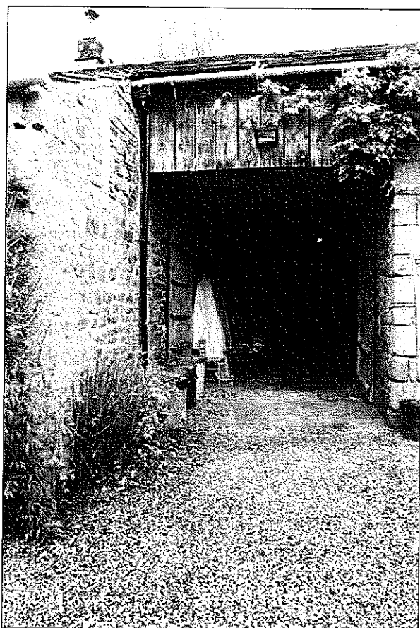
10 The stable joint by quoins of right wall of porch shows it is an addition
