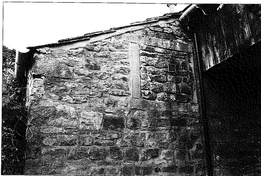
19 Northeast elevation showing blocked hayloft window and quoins of barn porch
