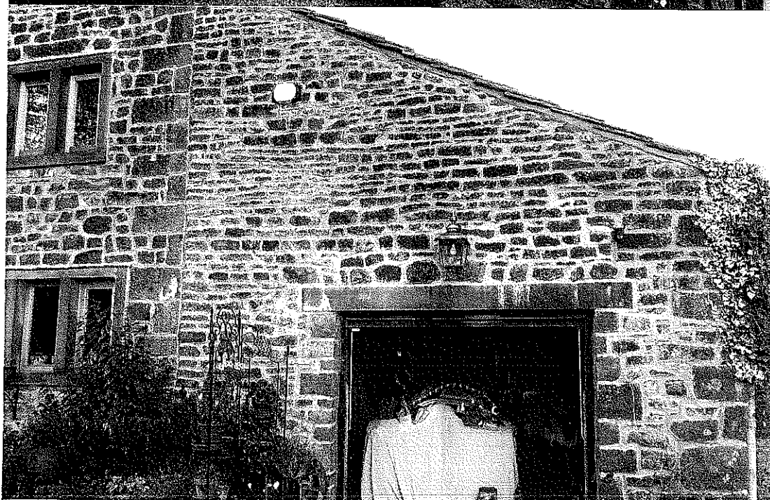
Photo 5 Existing Garage for Proposed Conversion
