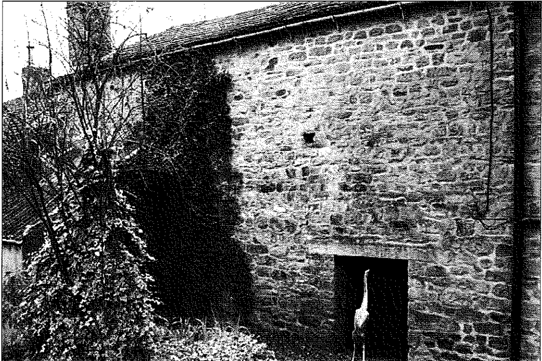
11 Rear (northwest facing) elevation of the barn showing door to threshing floor
