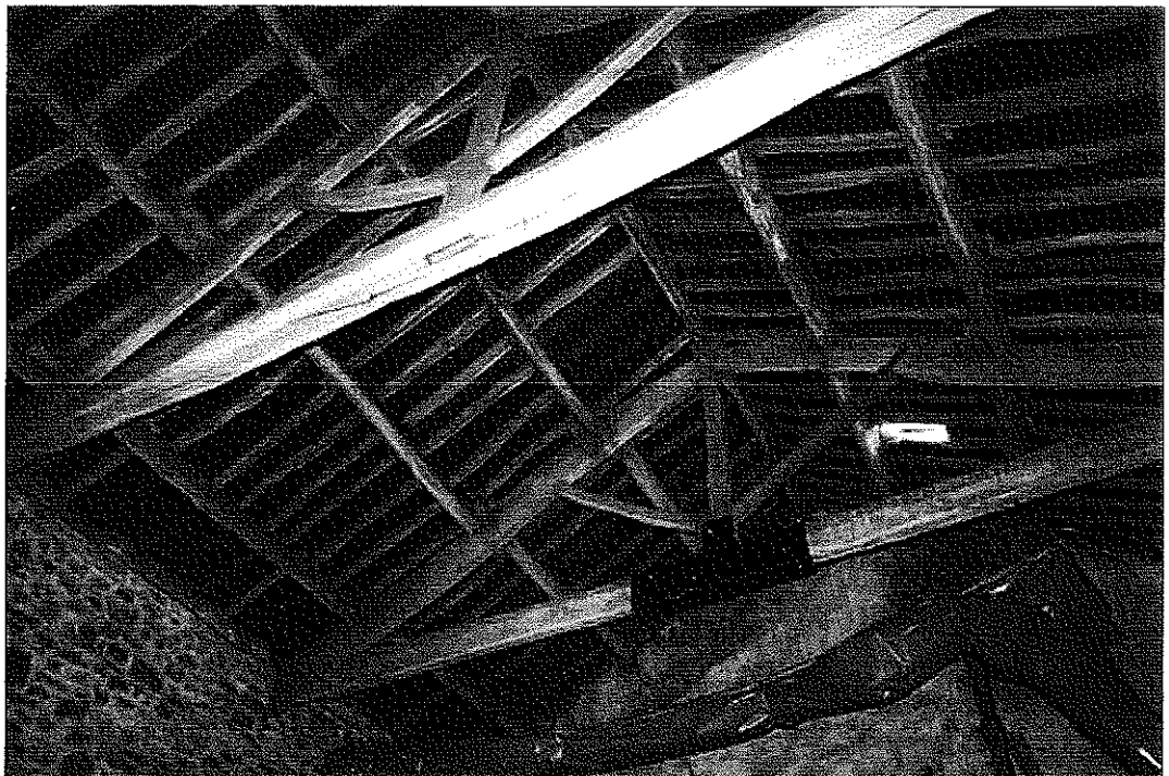
12 Kingpost roof trusses above the barn
