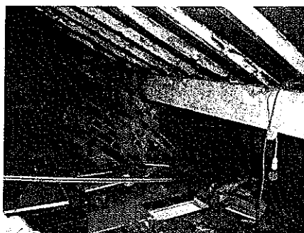
Figure 5: house roof void
