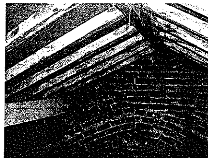
Figure 6: house roof void
