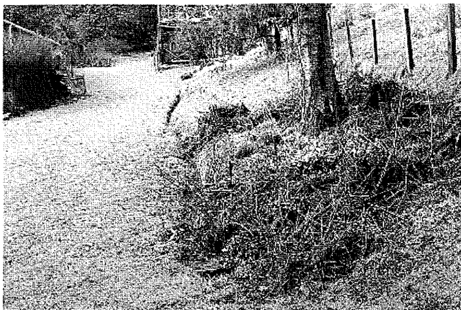
Catchment B existing overflow channel
