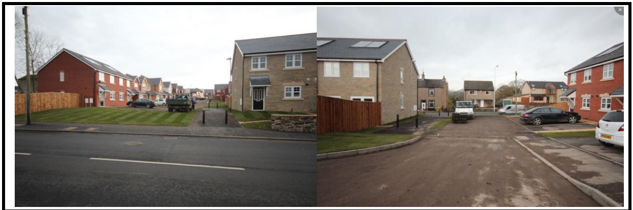
View of non car route from phase 1 to Whalley Road
