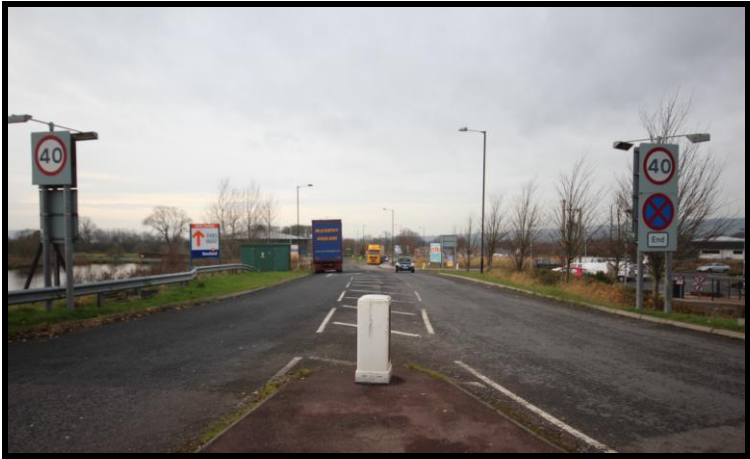
View along main access road from roundabout
