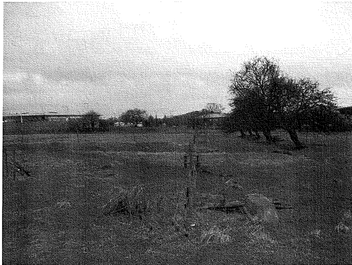
Photo 7 – S area of site, looking S with "Printworks" new office building (centre) to S of site (on site of infilled mill ponds) and petrol station (left).
