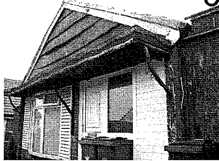
Figure 2: front (south) elevation
