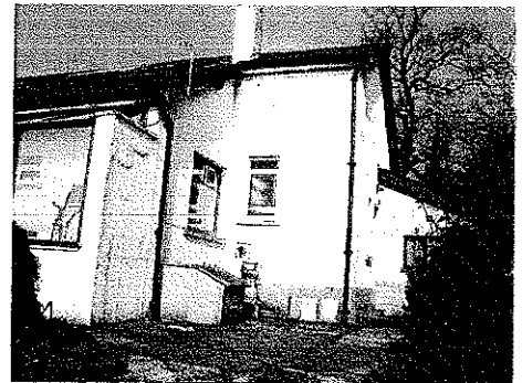
Figure 4: rear elevation, garage rear wall
