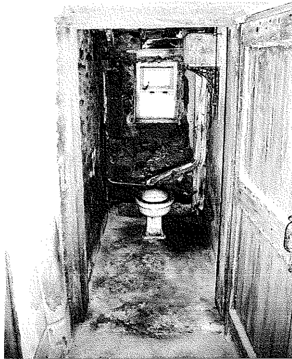
Image 16 - Original stone door surround and wrought iron ironmongery to WC
