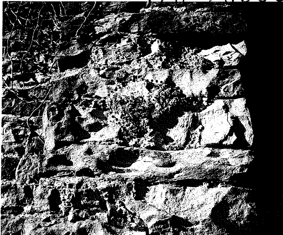
Image 18 - Evidence of original roughcast lime render to barn
