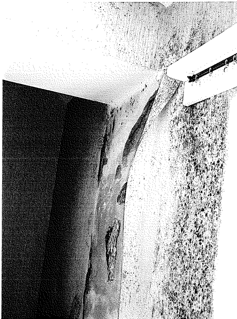
Image 31 – Evidence of serious dampness and condensation at first floor level
