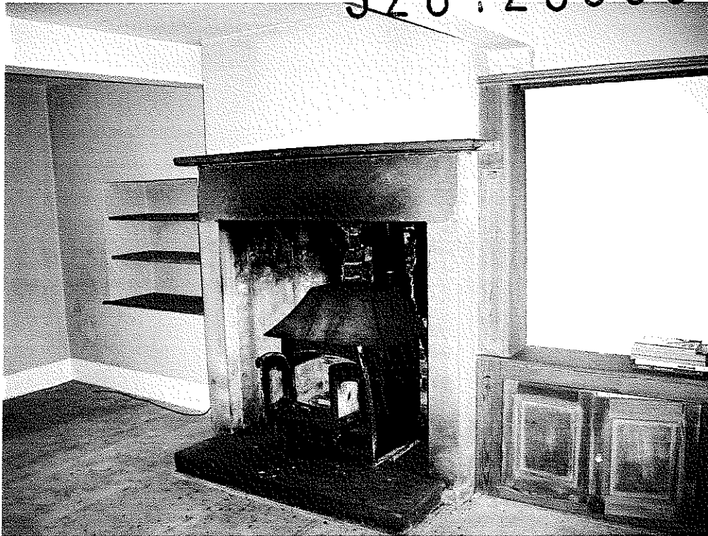
Image 14 - Plain stone fireplace (with brick backing) to Sitting Room
