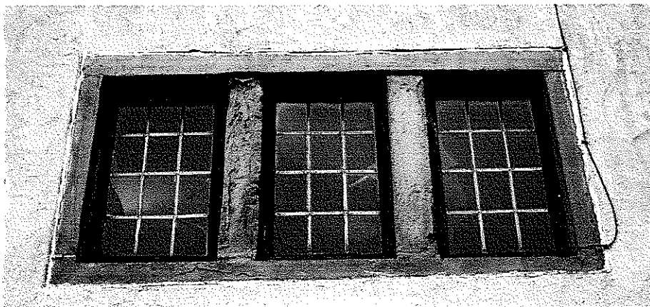
Image 2 - 3-bay stone square cut mullion window with metal framed leaded lights to Bedroom 2
