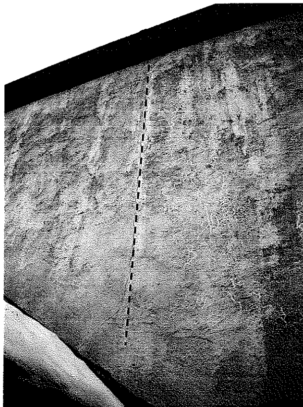
Image 12 - Assumed straight joint to front elevation
