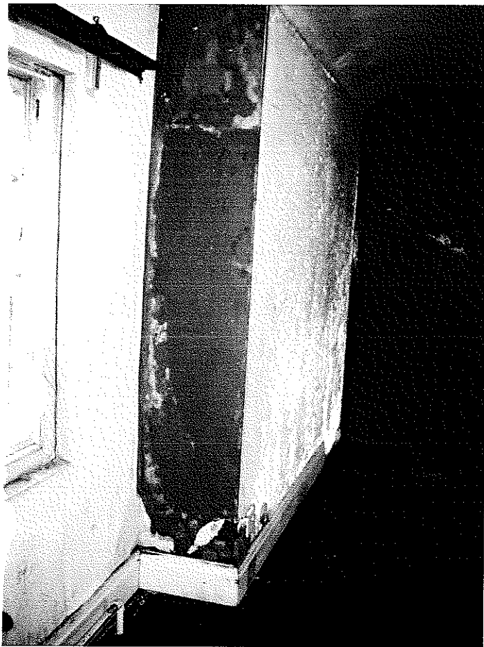
Image 25 - Water damage due to leaking junction at rear chimney/roof junction
