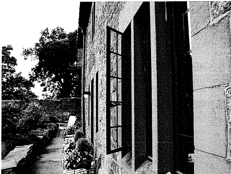
Image 23 - New metal opening casements, note neoprene gaskets and security to hardware
