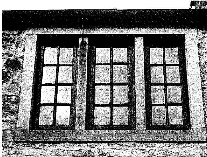
Image 3 - modern timber casements and saw cut stone surround to Bedroom 5
