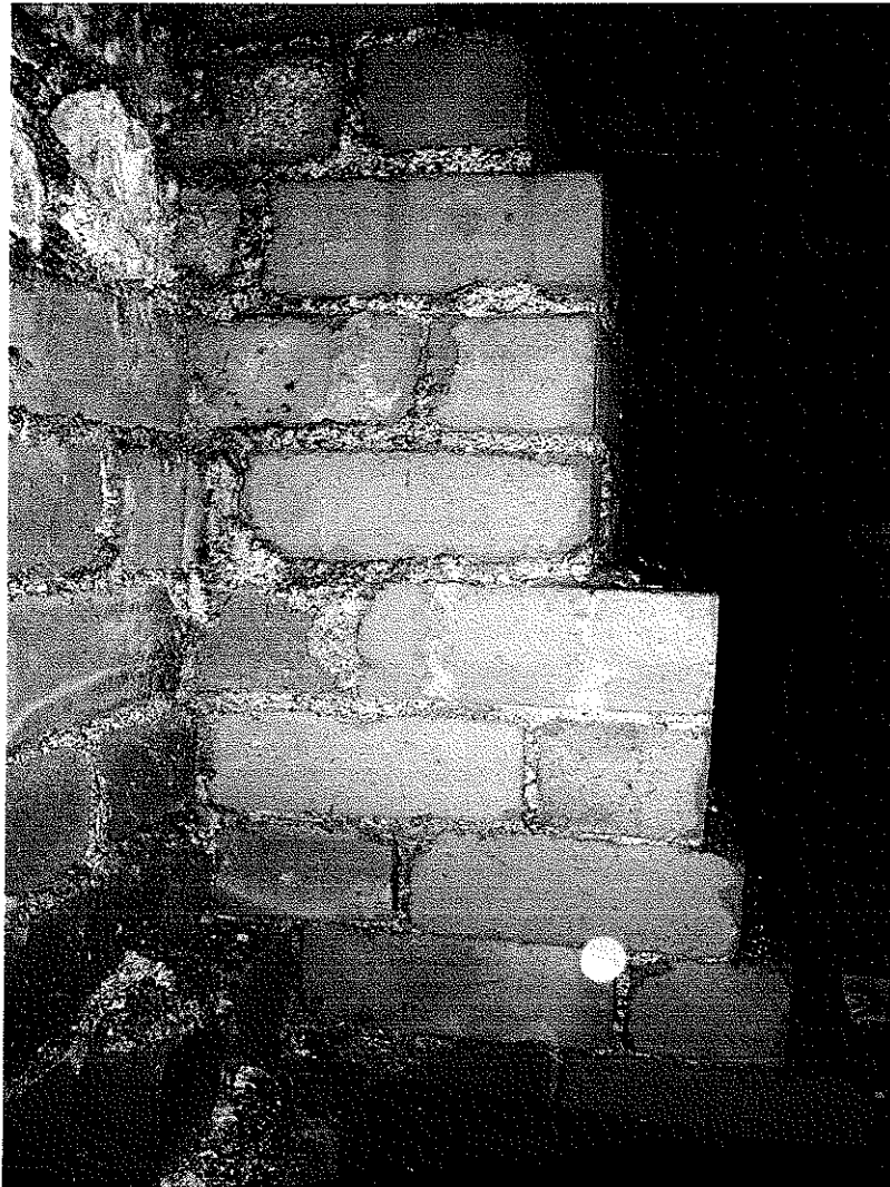
Image 13: Mid 20th C brick chimney in roof void above Bedroom 4 (kitchen)
