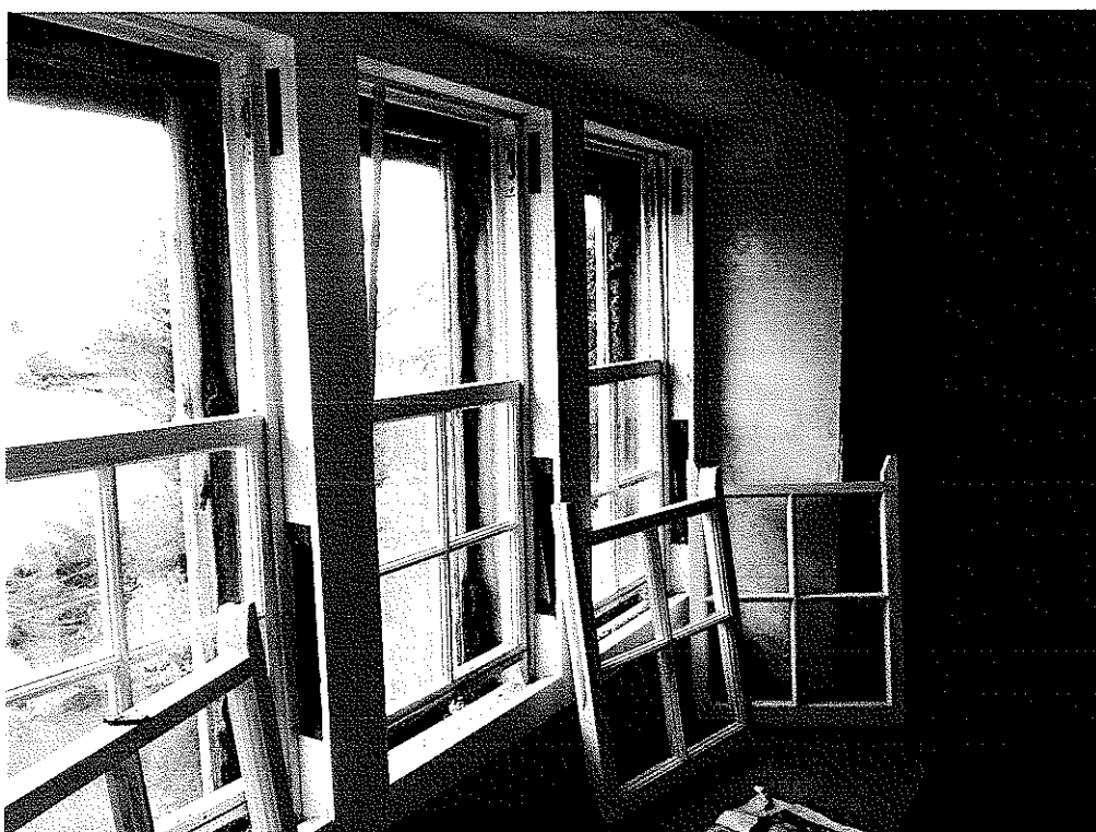
Image 19 - Current condition of timber sliding sash windows to rear elevation (Bedroom 1)
