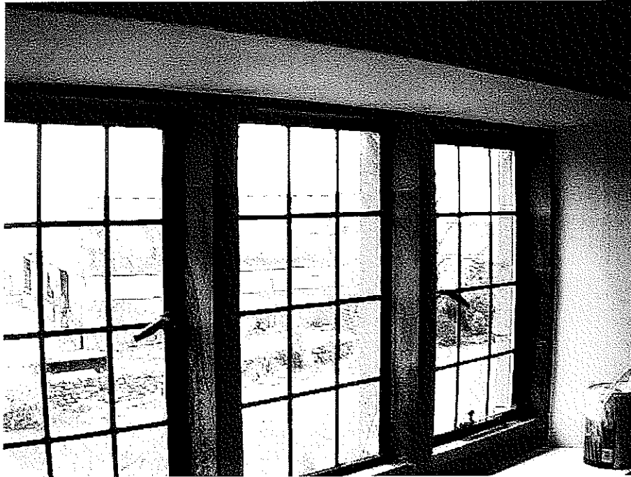
Image 22 - New fixed casement metal windows to a similar window detail in Northumberland
