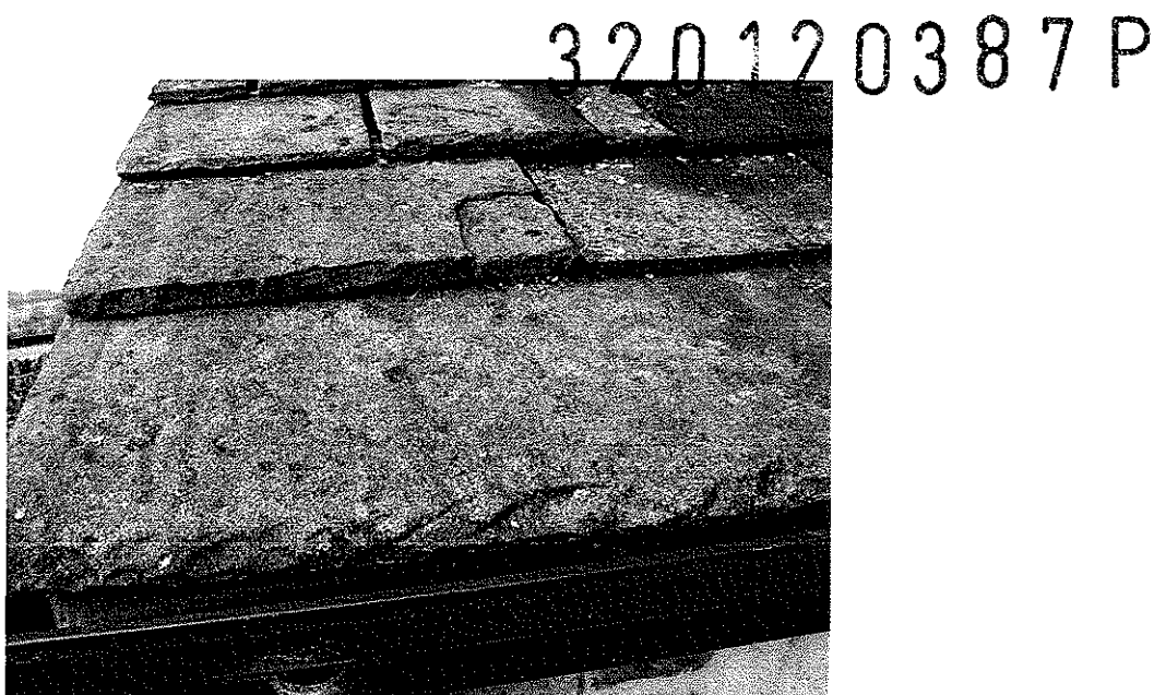
PI. 2 The above photograph shows samples of the natural grey slate that would be used to finish the proposed extension roof, which would match the existing house.
