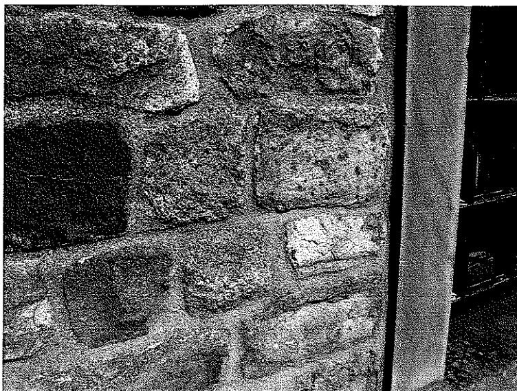
PI.1 The above photograph shows samples of the reclaimed natural stone that would be used to clad the external walls of the proposed extension and the dressed stone for the surrounds – all to match the existing house.
