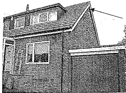
Figure 2: garage and S gable wall
