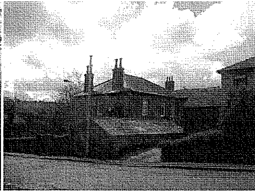
East/North elevation and outbuilding
