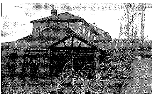
Outbuilding South elevation
