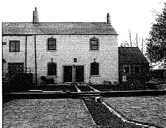
Image 2. No.1 Edisford Hall Cottages Front (please note that the proposed garage / storage block is approximately 20 m away from the cottage to the right hand side of the property).
