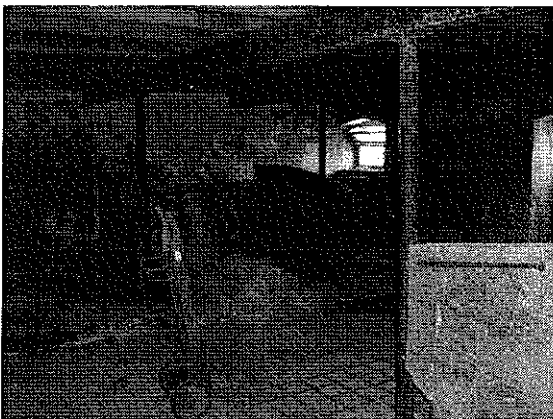
Shippon with hay loft on metal columns
