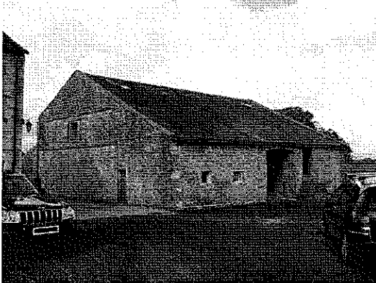
South elevation with wagon entrance
