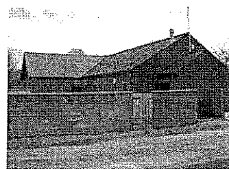
Figure 3: rear (west) elevation
