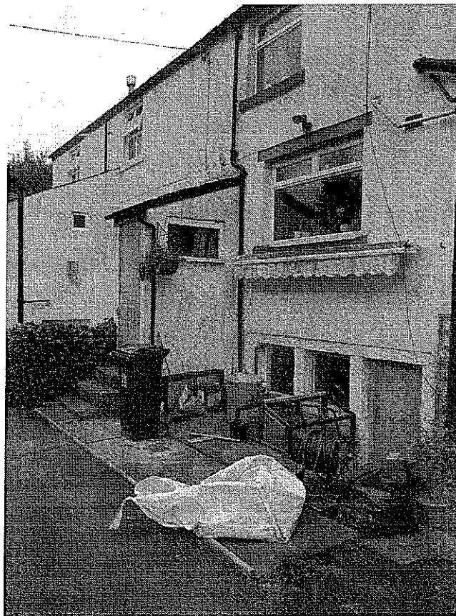
47 Avenue Road, Rear Addition
