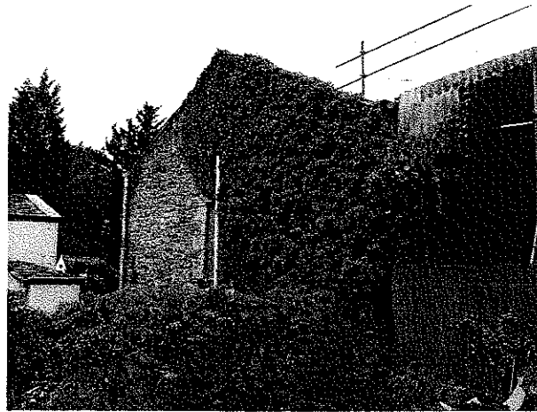
PL 11 Vegetation growth potentially concealing defects / breaking down existing wall stability
