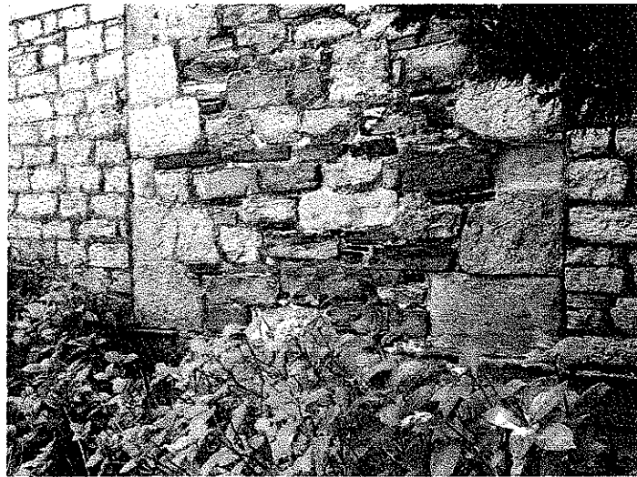
PL. 9 Re-point/build section of external wall.
