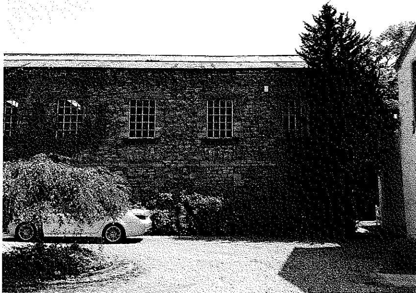
PL. 2 View of South West structural wall from courtyard
