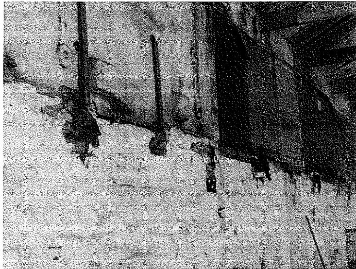
PL 17 Evidence of existing floor joist slots
