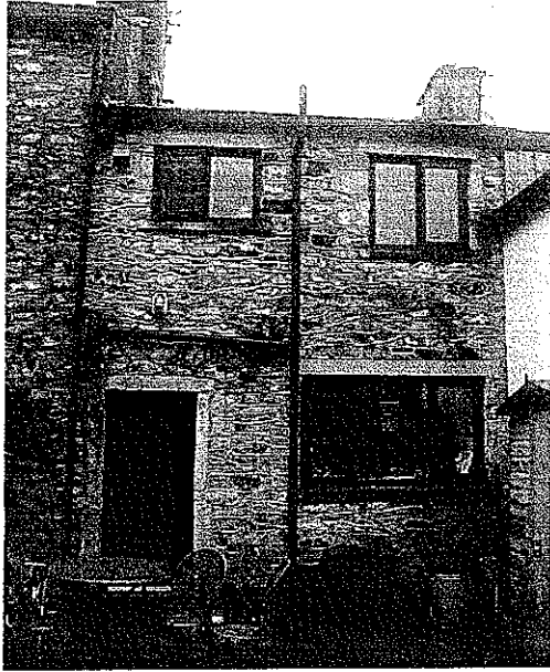
Rear elevation of cottage.
