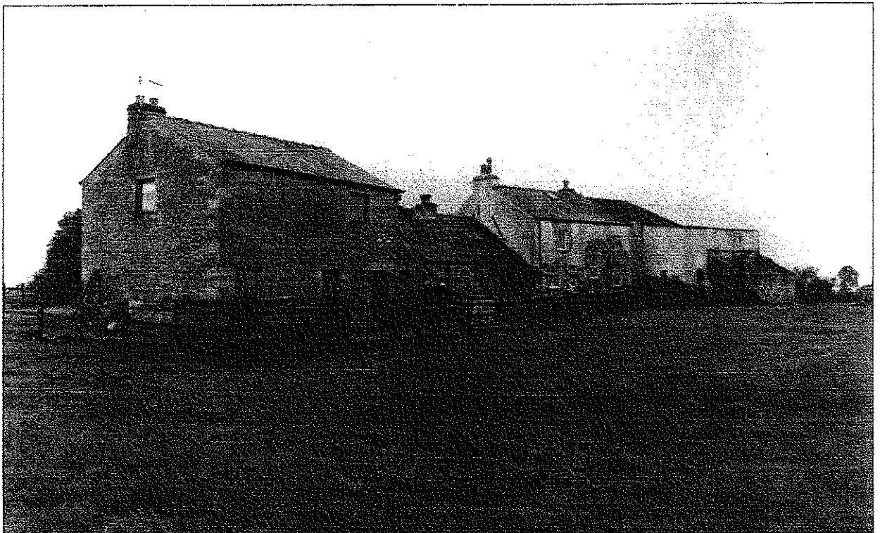
Photo 4: General view of Huckle Ing, from the north-east
