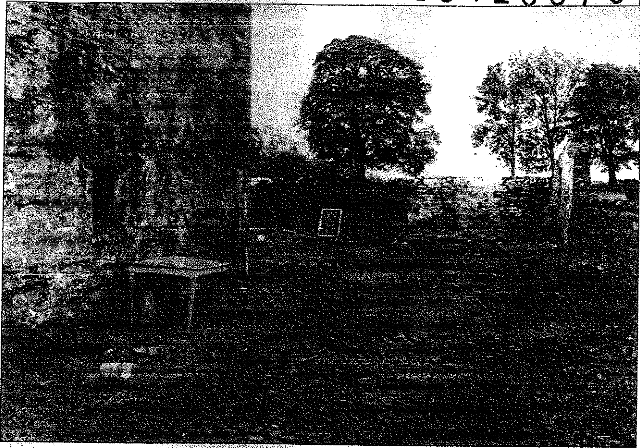
Photo 9: Cobbled yard next to west gable, and remains of outbuilding
