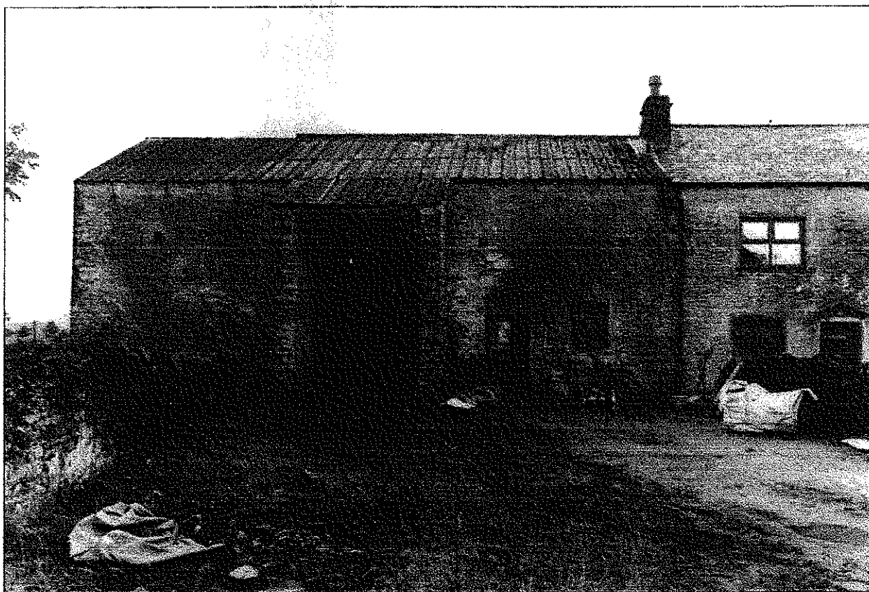
Photo 2: Front elevation of the barn
