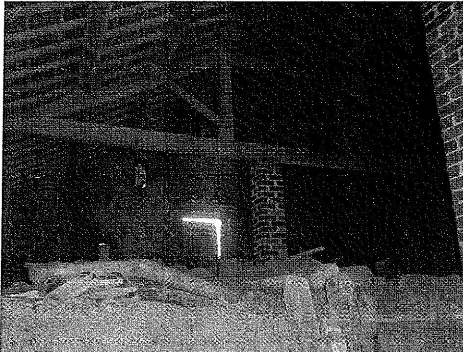
Internal shot of redundant building (queen post trusses to be retained)
