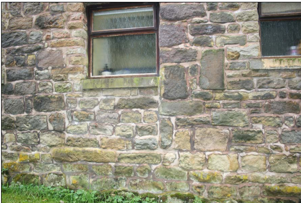
15. Evidence of rebuilding or blocked opening on rear wall between second and third bays
