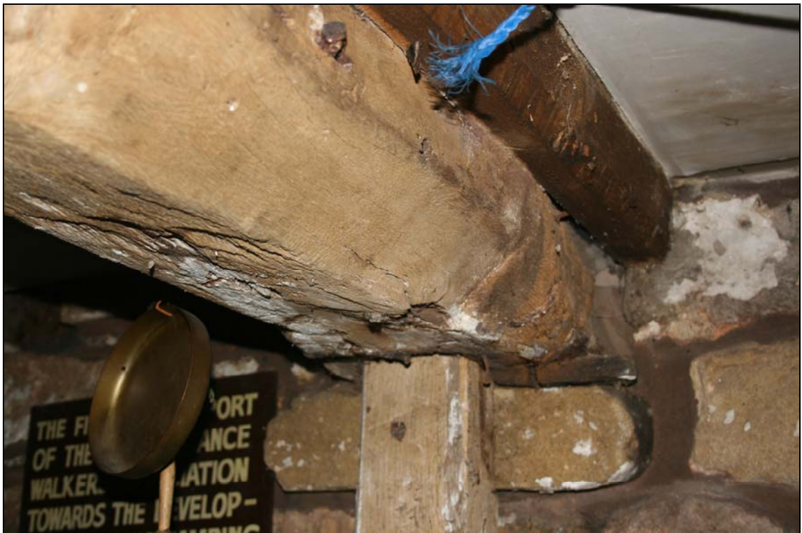
17. Detail of chamfered and stopped beam
