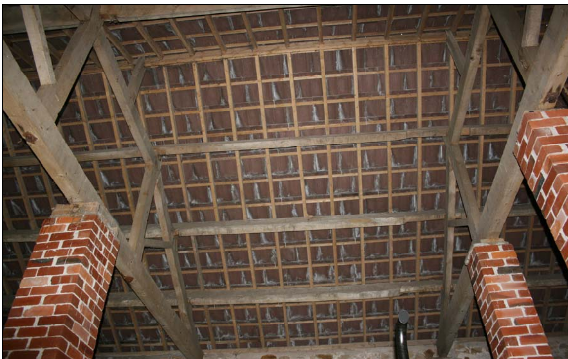
24. Trusses flanking threshing bay
