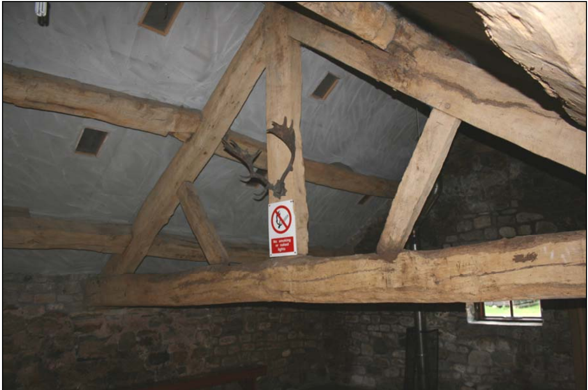
18. Kingpost roof truss over camping barn
