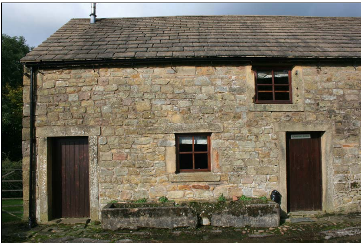
12. Detail of camping barn showing 19 th century window and door surrounds with exception of ground floor window whose jambs seem earlier, probably from two-light mullioned window
