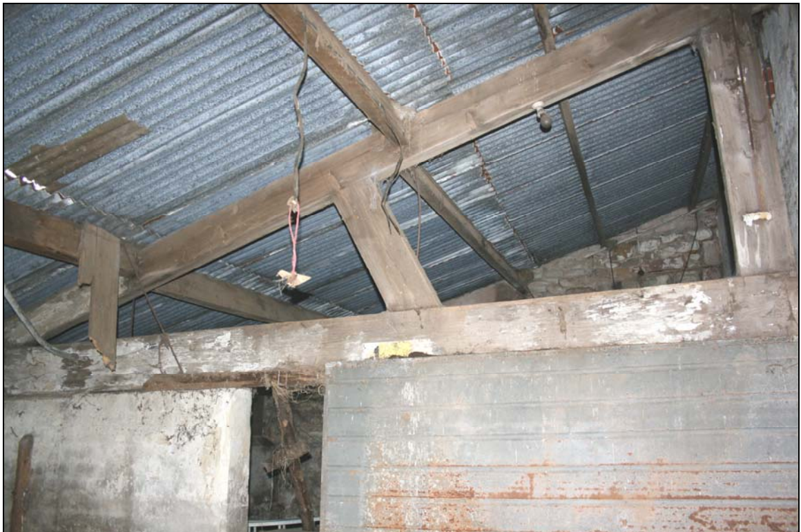
35. Half-truss within the garage
