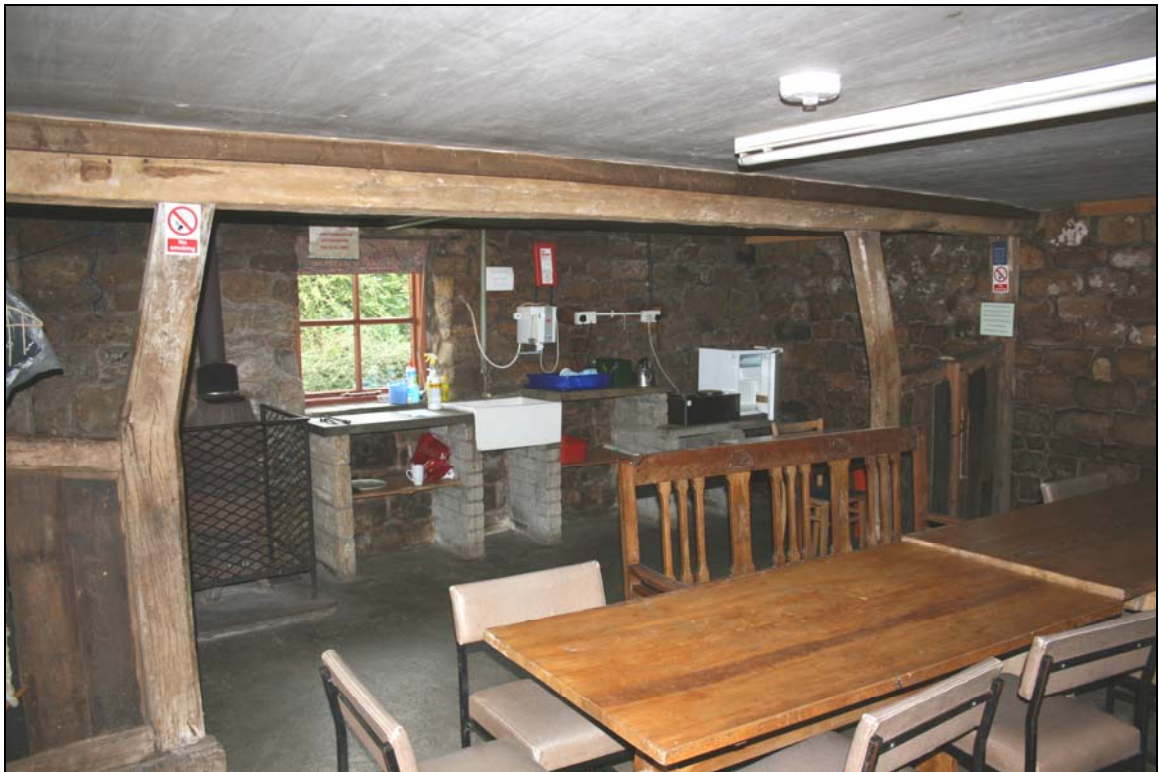
16. Interior of camping barn showing stall posts relocated beneath beam
