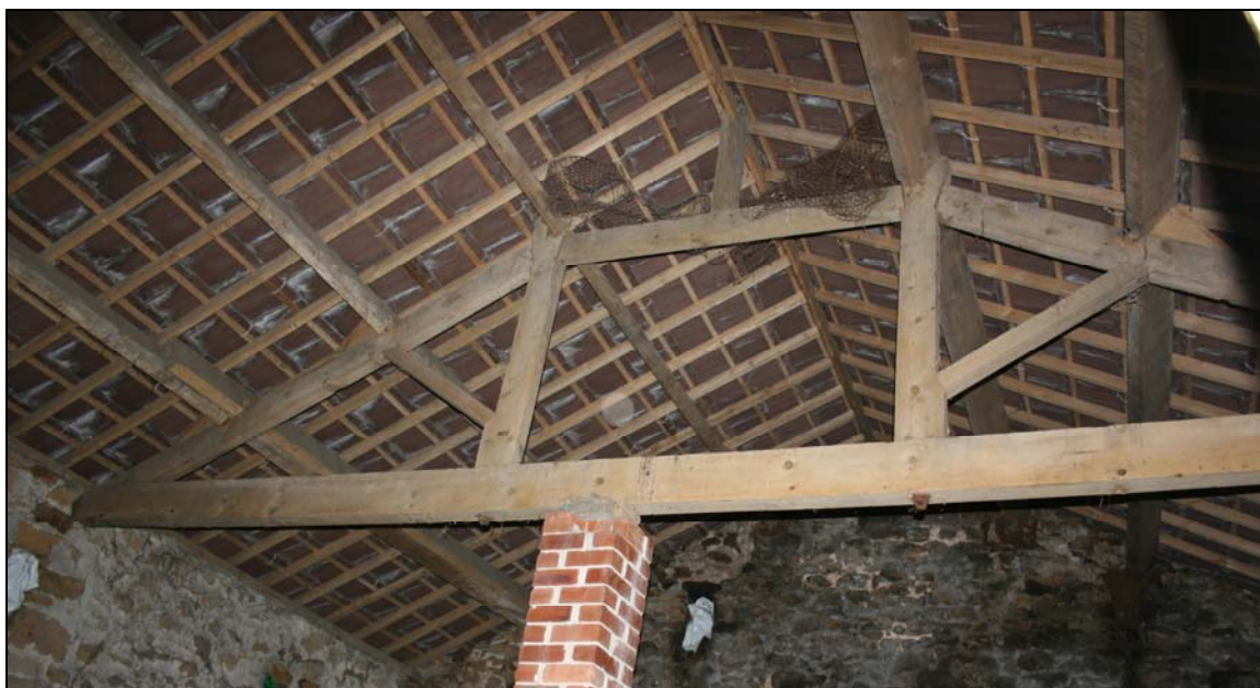
23. Truss above shippon and hayloft
