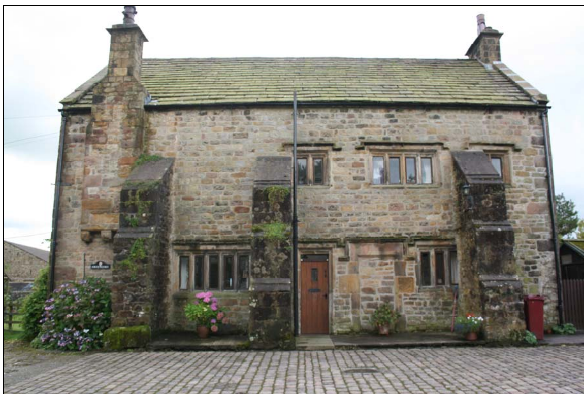
8. North elevation: blocked entrance may itself have been an insertion
