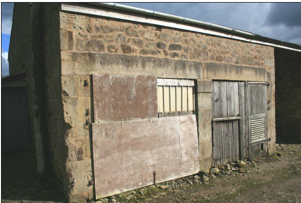
28. Former cartshed entrances; gudgeon pins for doors remain in situ
