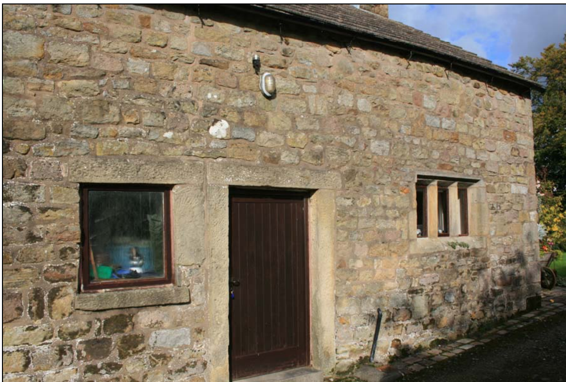
11. 19 th century door and window and 17 th century window and mullioned window of cottage
