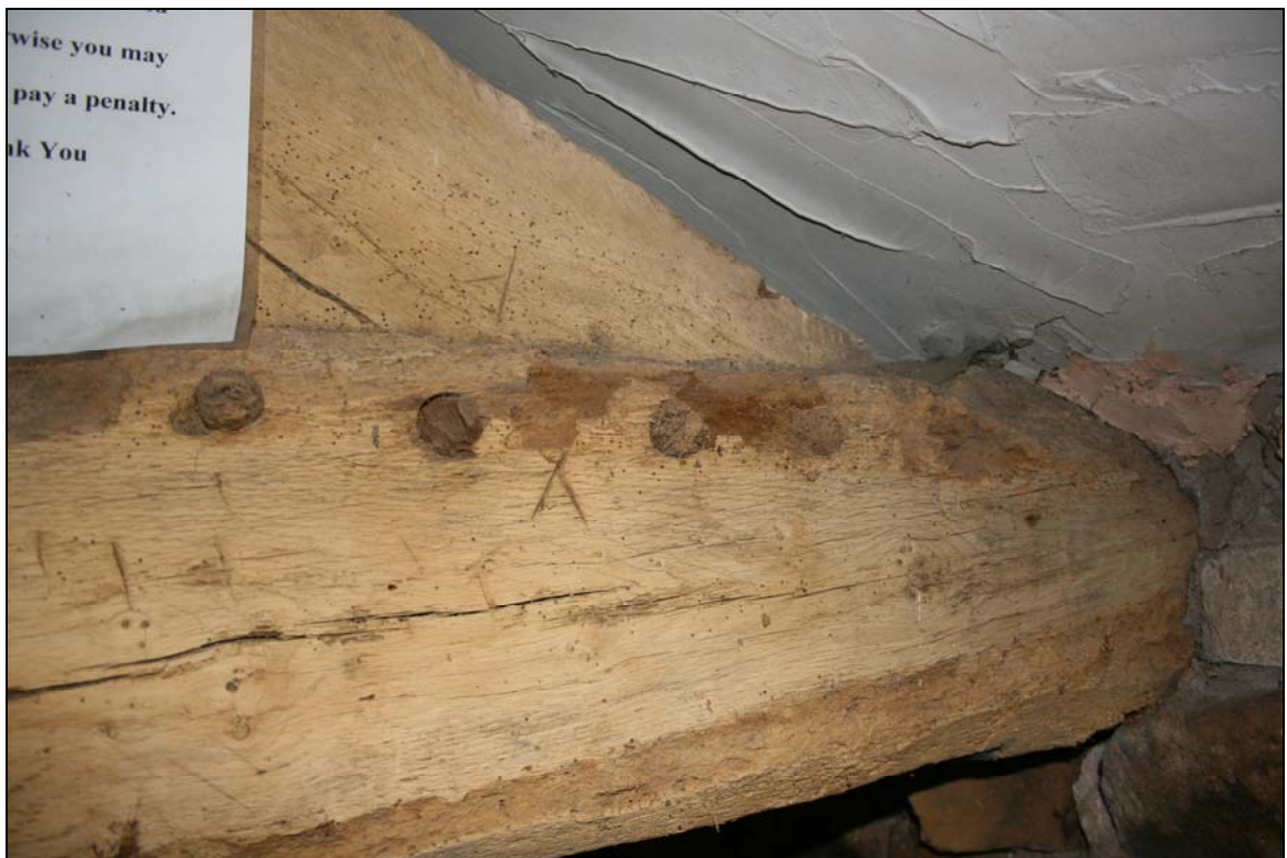
19. Assembly marks on east face of truss
