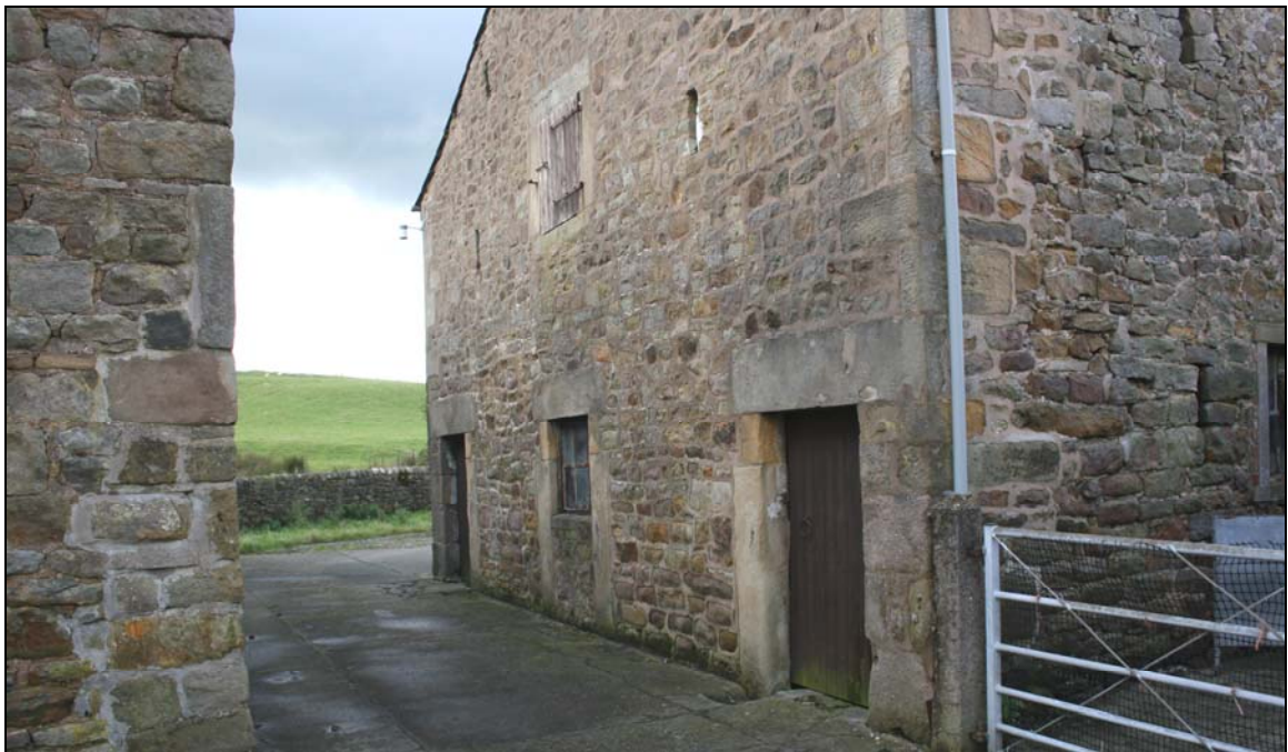
25. South gable showing three-door arrangement of shippon
