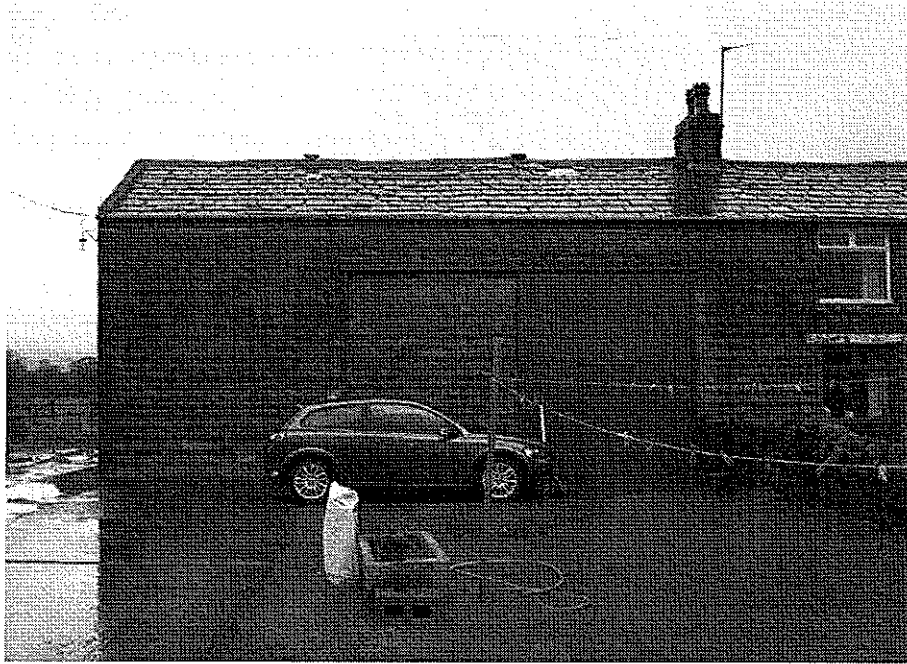
Photo 2 – Existing South Elevation (Front)
