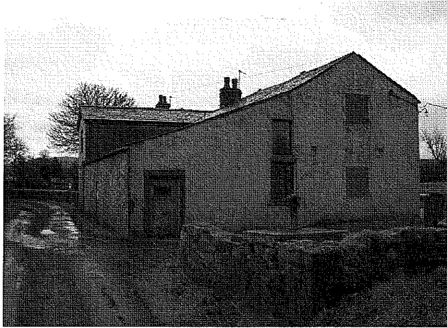
Photo 1 : West Elevation – As existing
