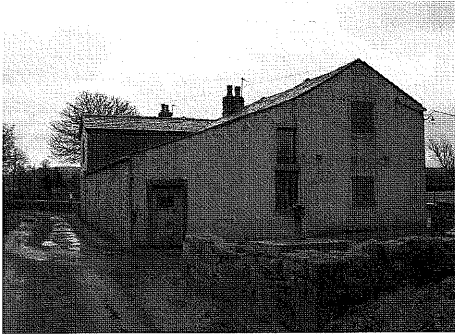
Photo 3 – Existing West Elevation (Side)
