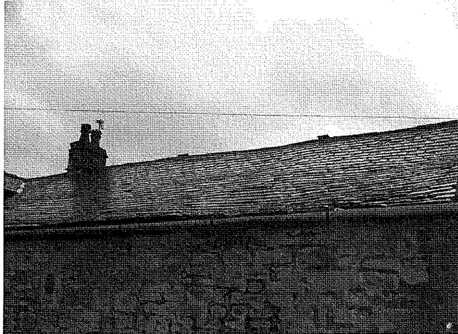
Photo 14 – Roof Covering – Main Barn/ Shippon, North Face
