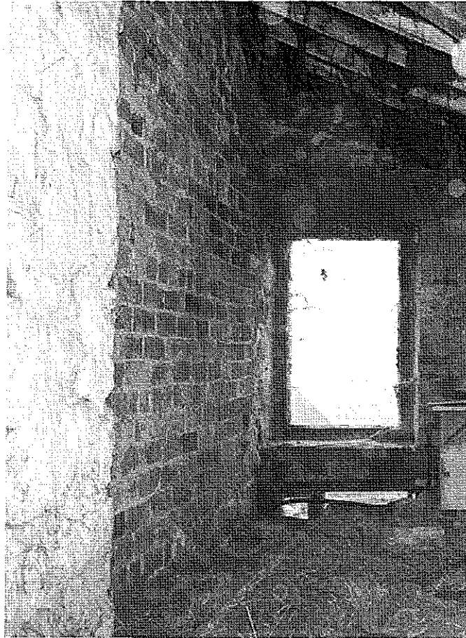
Photos 16 – Internal brick wall
