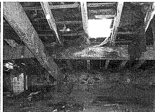
Photo 13 – Roof Timbers – Shippon
