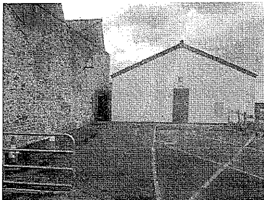
Images of the wall after lean to building removed, wall washed down and re-pointed in lime mortar
