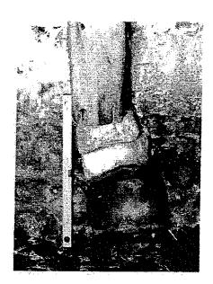
The other three plinths appear to be reasonably plumb and stable, though the cruck blades are not vertical (see section 2.9) In view of the condition of the others though it makes sense to treat them all similarly and ensure that they are well restrained
