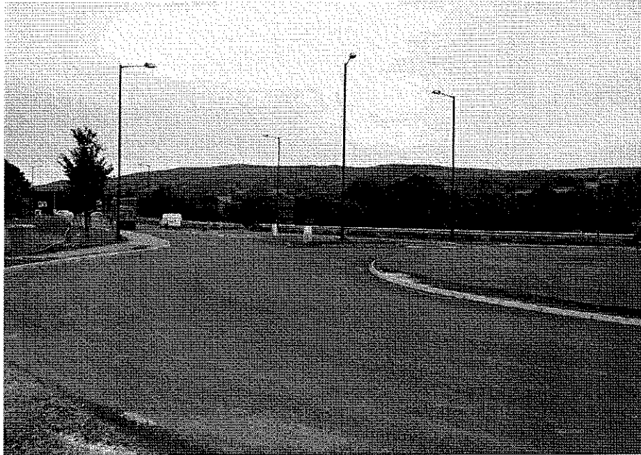
Existing Infrastructure off A59
