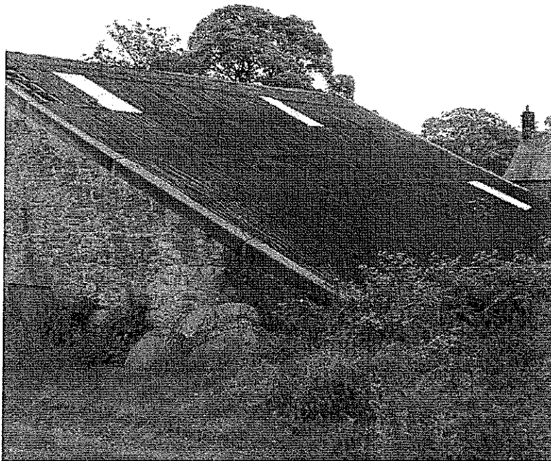
Plate 2 ~ Undulating roof finishes to rear pitch
