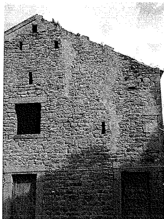
Plate 10 – 'Re-pointed' masonry cracking
