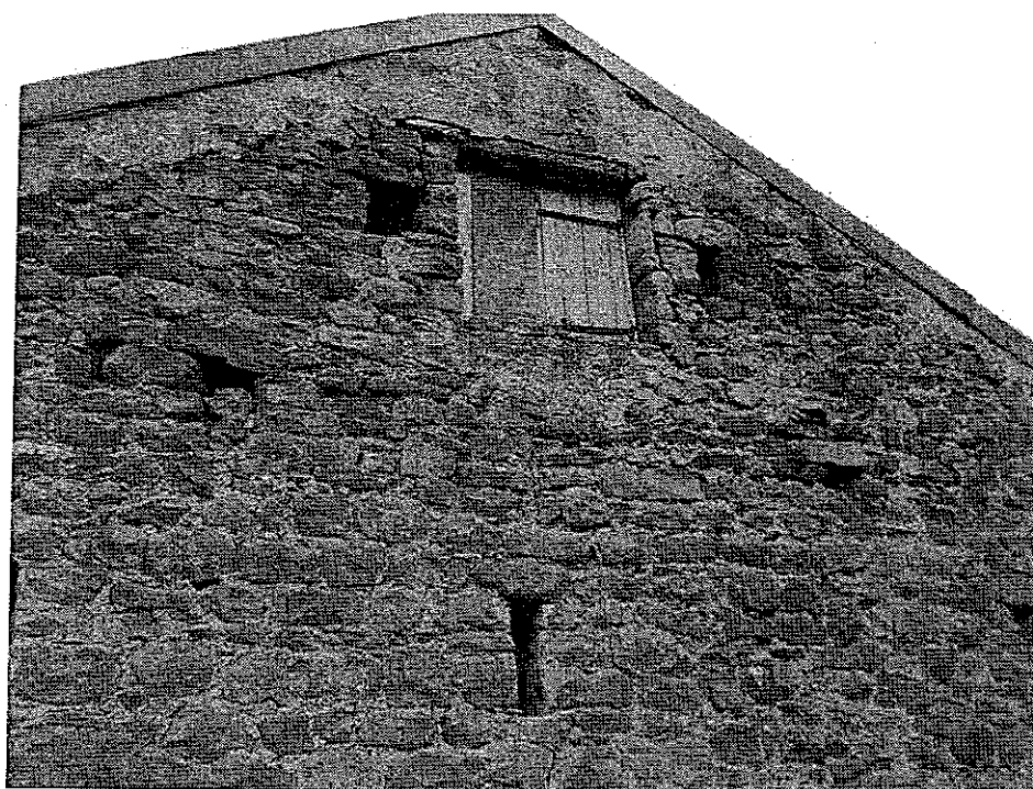
Plate 3 – Weathered mortar to North gable apex
