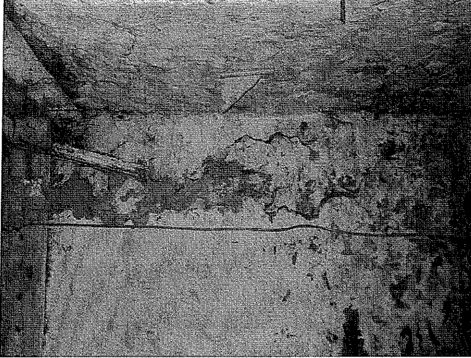
Plate 36 — Vertical crack, damp penetration to applied Shippon wall finishes
