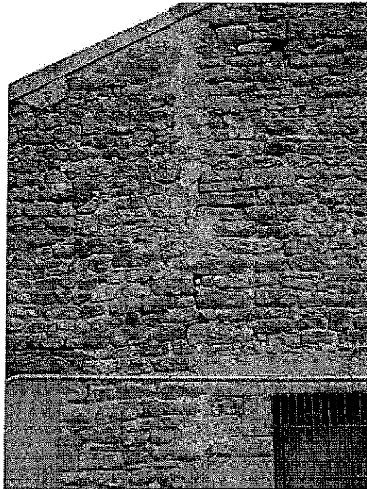
Plate 11 – 'Re-pointed' masonry cracking ('Shippon')
