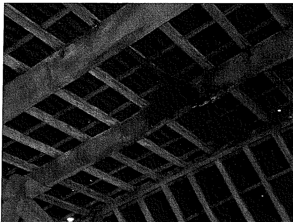
Plate 17 – Damp and rot to purlin
