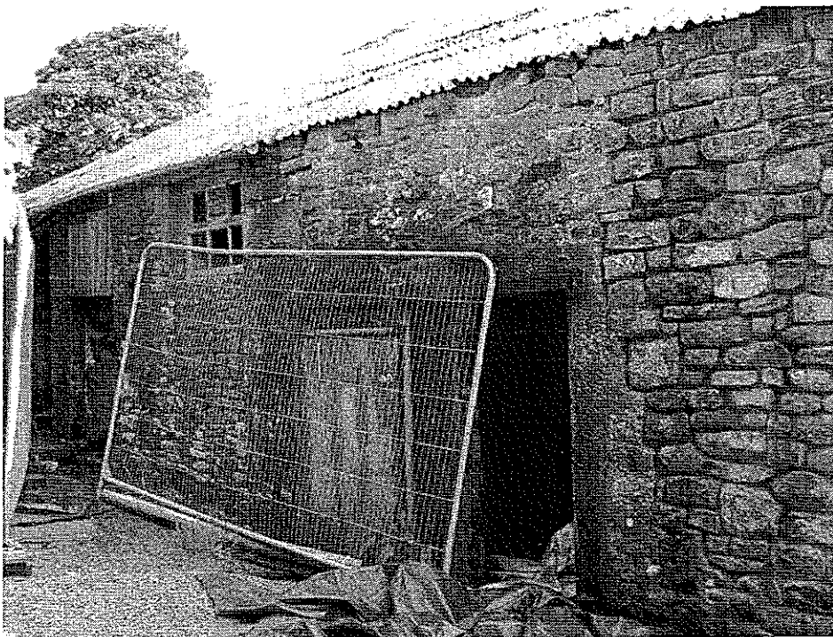
Plate 14 – Weathering to West (rear) Elevation
