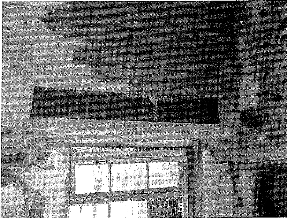
Plate 21 – Pre-stressed concrete lintel replacement
