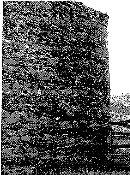
Plate 7 – Water staining and vegetation growth
