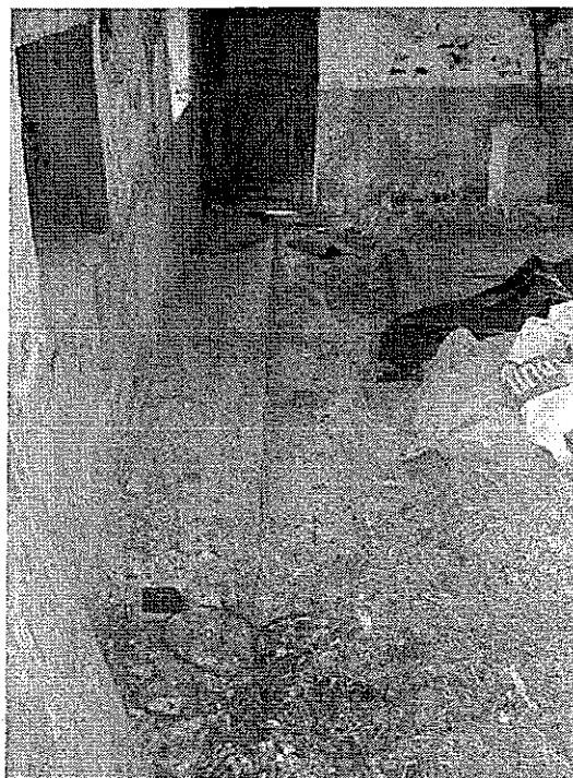
Plate 24 – Lower lying concrete ground bearing slab
