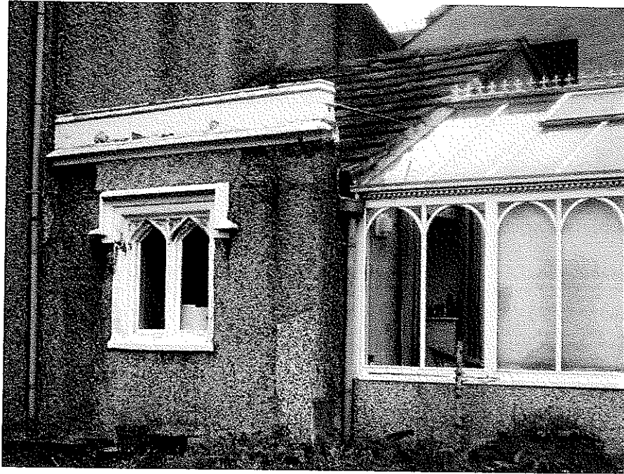
Photo 2 – Showing Front of Kitchen Wall.
