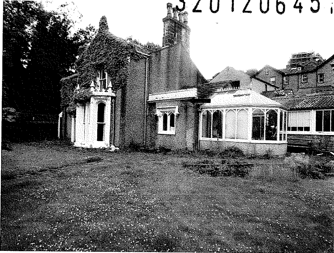
Photo 1- Front Elevation Stanworth House.
