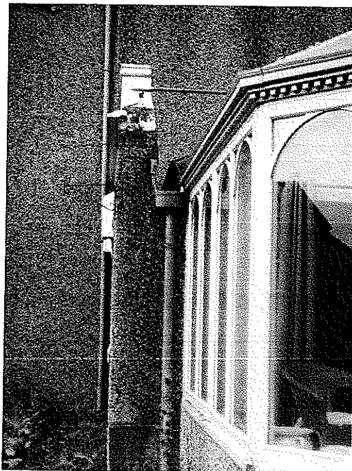
Photo 3- Showing Side View of Kitchen Wall and Valley Gutter.
