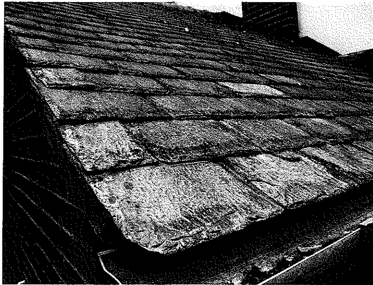
Pl. 3 The above photograph shows the kind of Westmoreland Green slates that would be used to finish the proposed extension roof, which would match the existing house.
