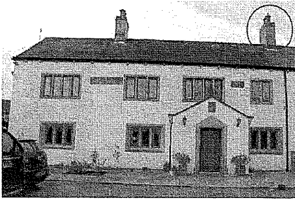
Photograph 4 NE elevation Edisford Hall Farmhouse
