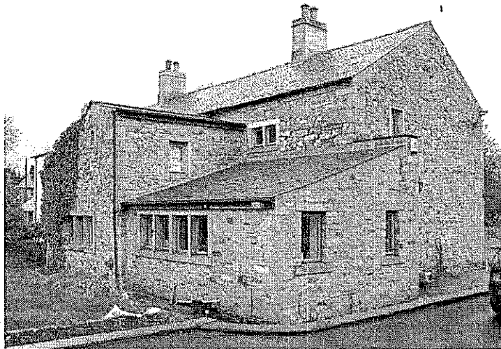
Photo 3: View of the farmhouse from the south-west, showing 1984 extension in centre of picture and much altered historic wing to left.
