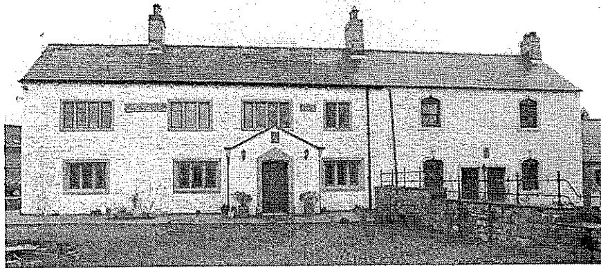
Photo 1: East elevation (rebuilt c.2006)
