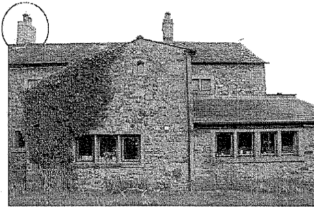
Photograph 5 SW elevation Edisford Hall Farmhouse
