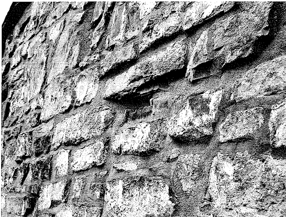
Figure 7: Irregular stonework to gable elevation
