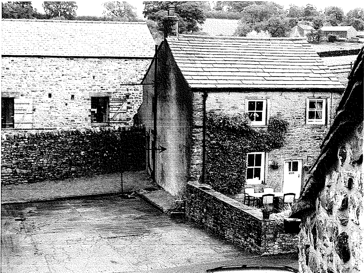
Figure 6: Cement roughcast render to gable elevation of 21 Brookside
