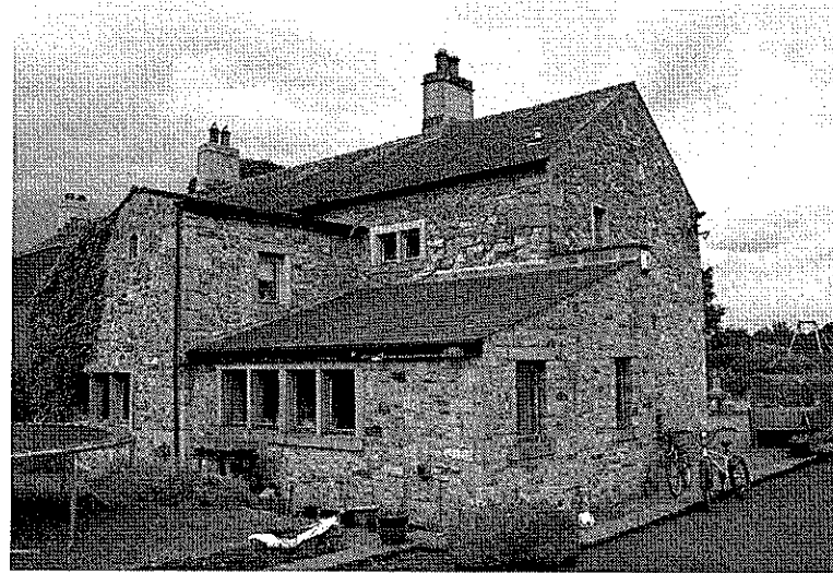
Photograph 1 View from the south side Edisford Hall Farmhouse
