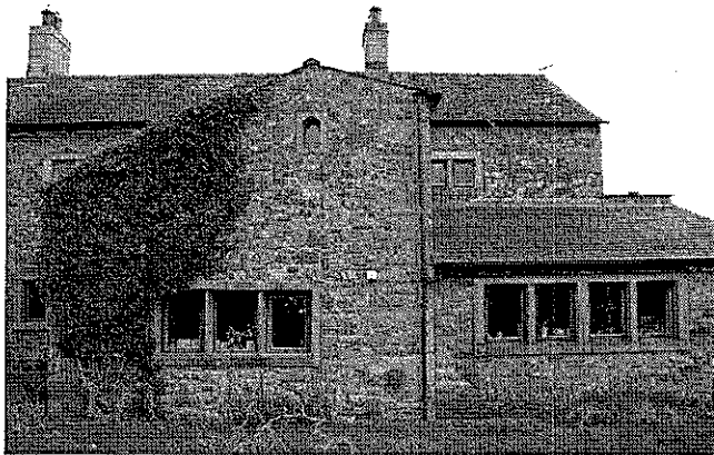
Photograph 5 SW elevation Edisford Hall Farmhouse
