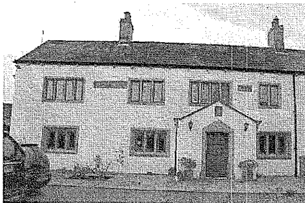
Photograph 4 NE elevation Edisford Hall Farmhouse
