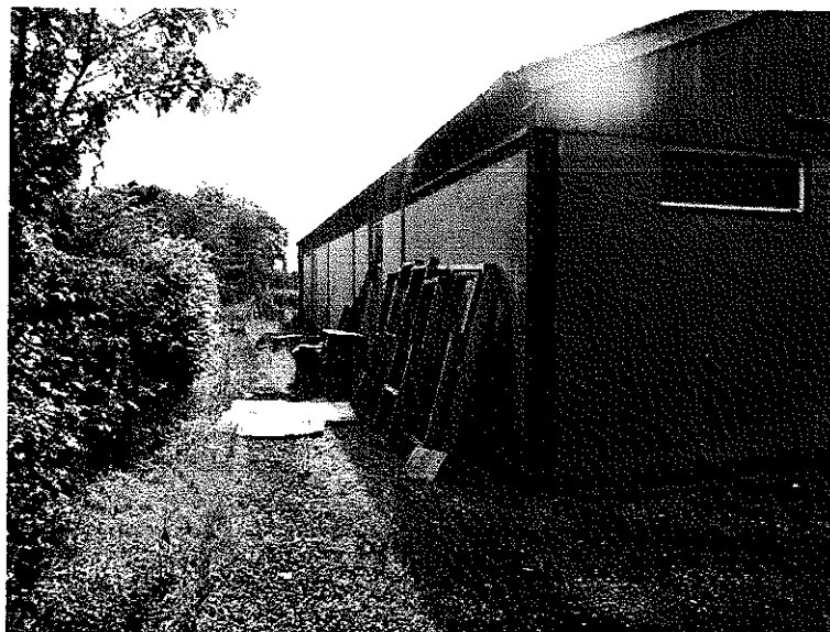
Pl. 10 Photograph showing the south eastern side of the outbuilding and the mature hedge boundary.
