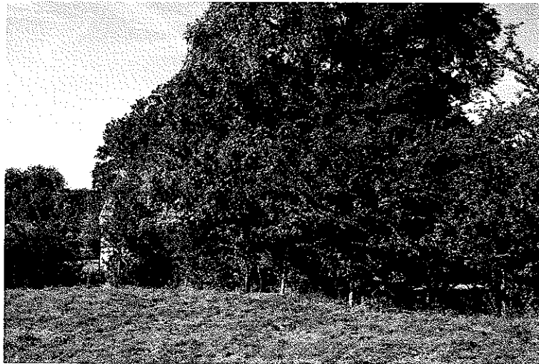
Pl. 9 Photograph showing the outbuilding from the adjacent field.
