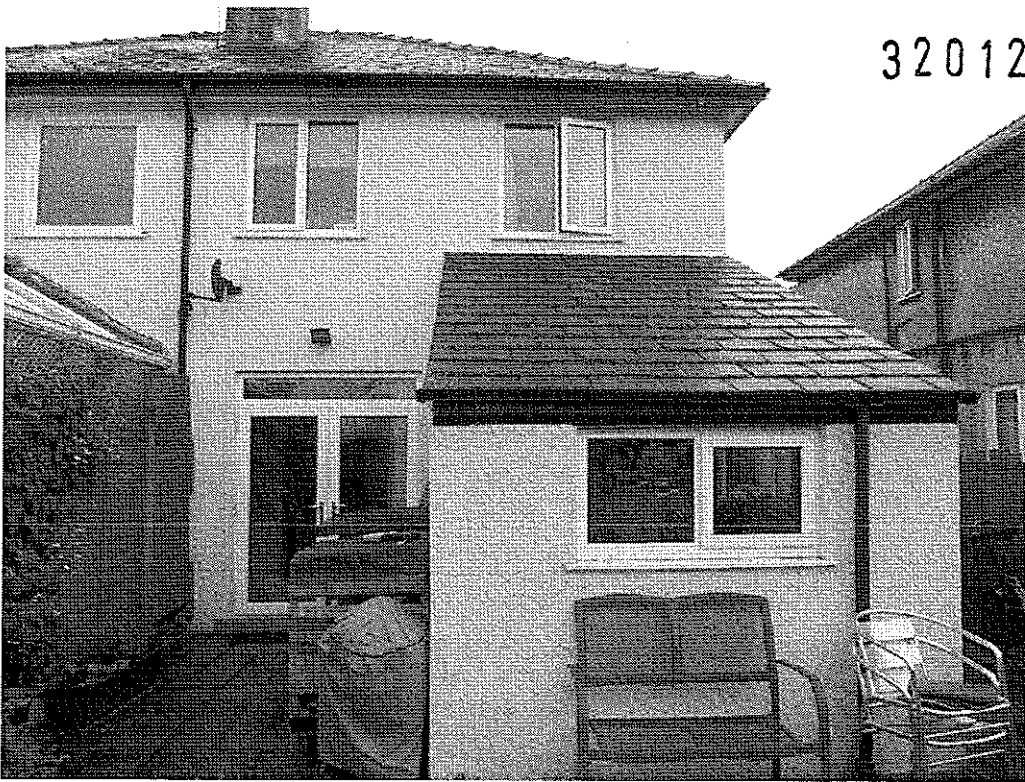
Photo 1 – View of existing rear extension (to be demolished)
