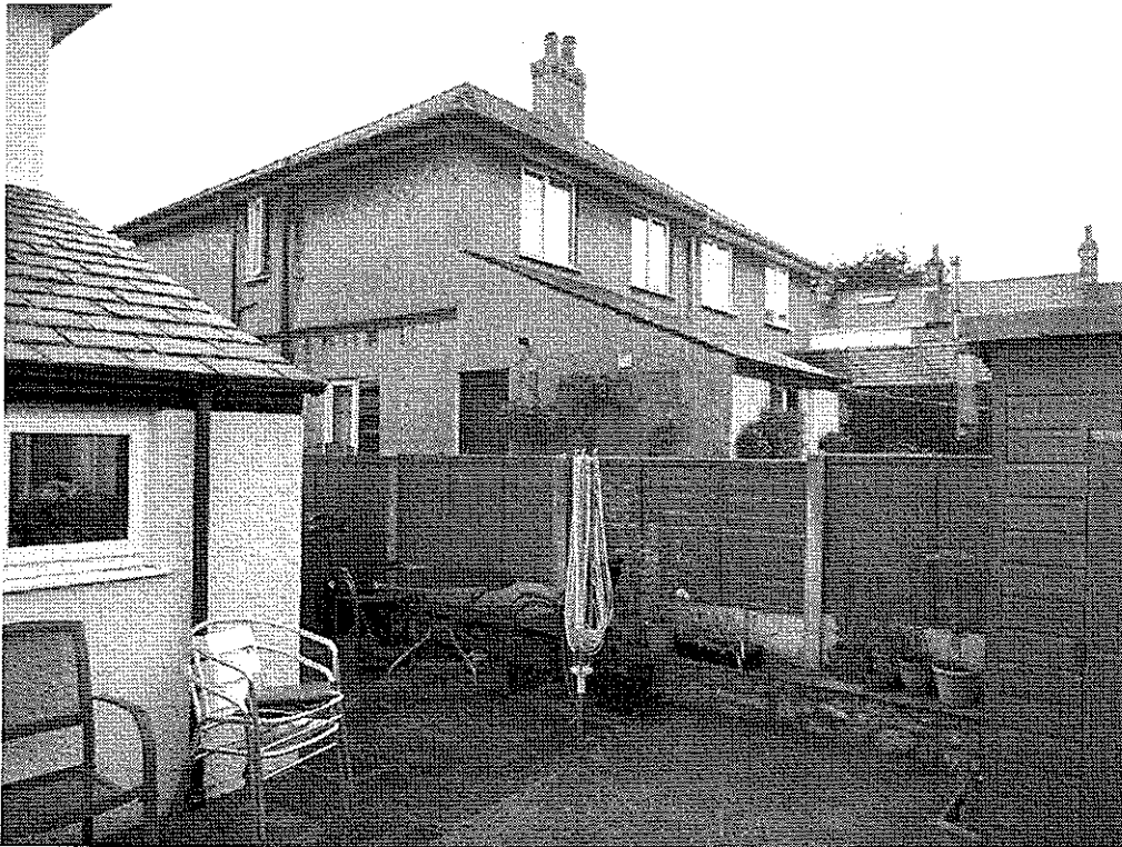
Photo 2 – View looking north west to adjacent property
