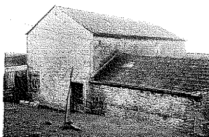
Figure 6: Barn C and Building 'B'
