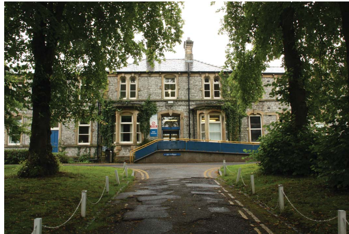
View of approach to existing hospital main entrance
