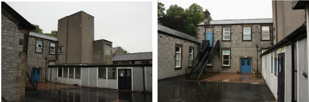
Views to rear of front building showing later additions:
