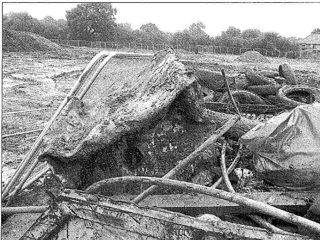
Plate 5 Photograph showing excavated septic tank
