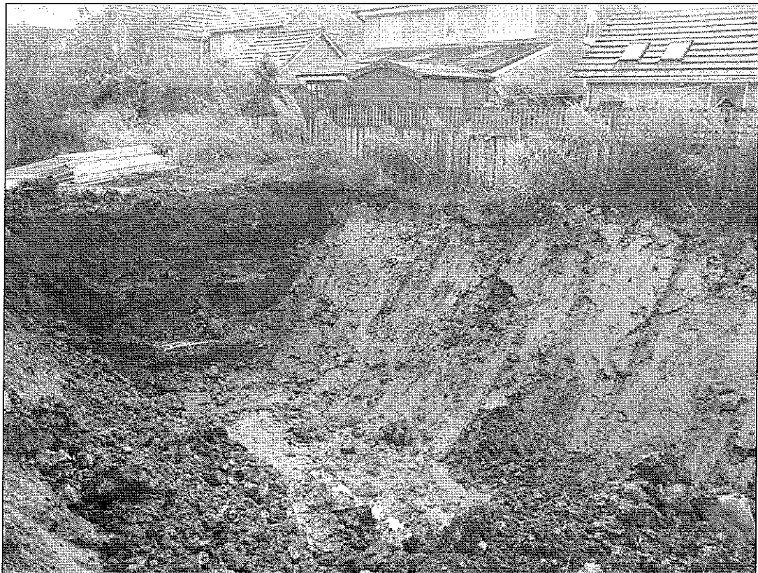
Plate 4 Photograph showing clay stank being emplaced within former cess pit
