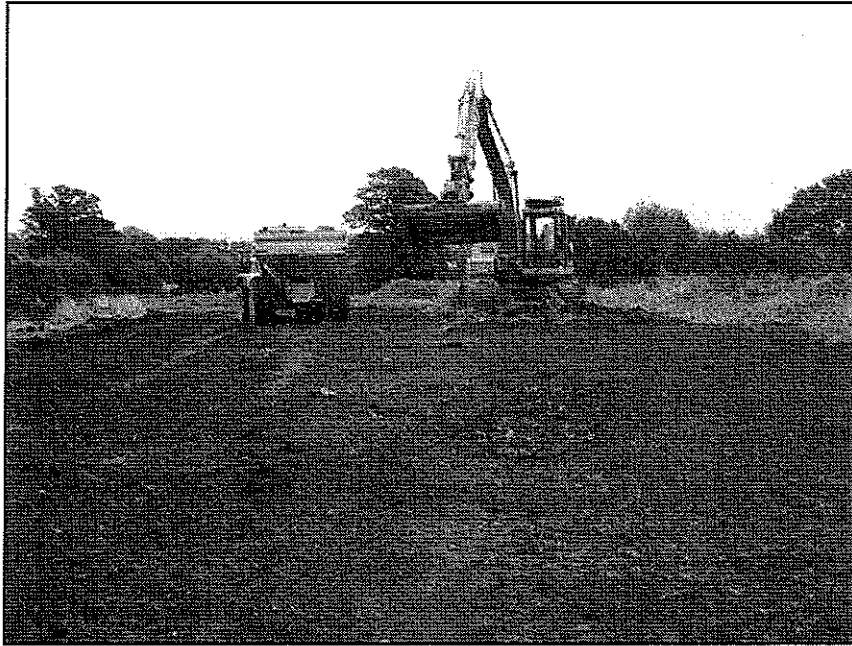
Photograph 3 showing vegetation stripping under supervision
