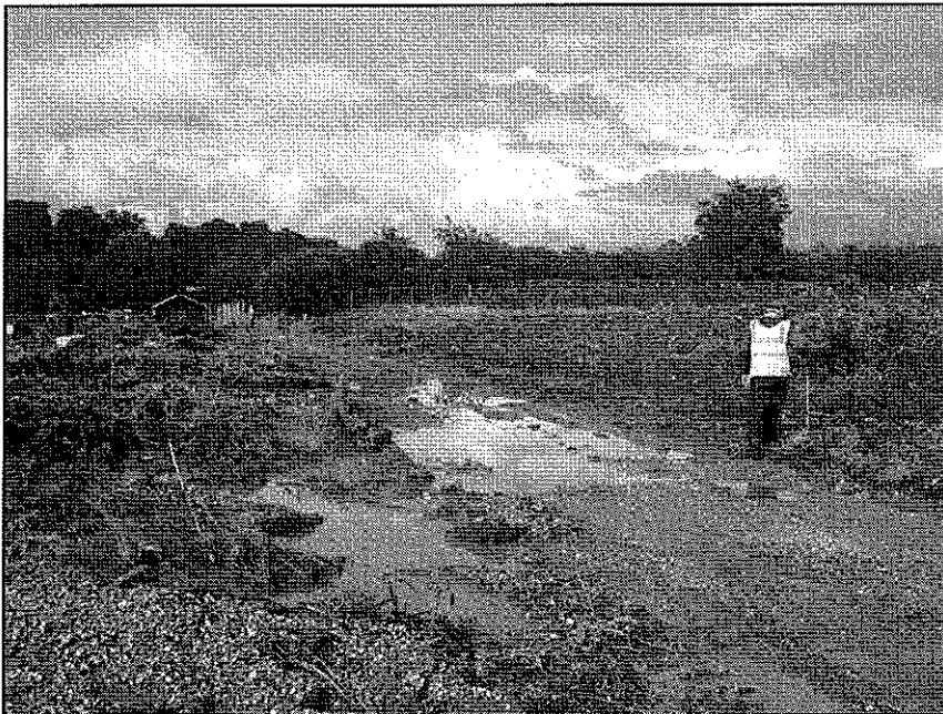
Photograph 6 showing the site of the removed hedgerow
