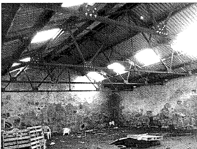
Photo 6. An internal view of the southern section of building showing the metal roof support frame and sky-lights
