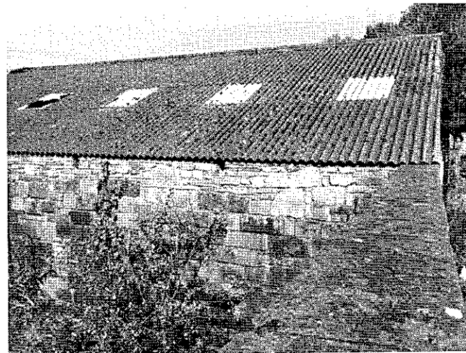
Photo 2. Detail of the southern section which will require removal to allow access to the site. Two small holes visible beneath the eaves presumably previous used for supporting timbers.
