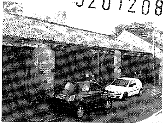
Photo 10. View towards the northern section of the building showing the two wooden sliding doors of the enclosed sections and where the building is attached to the adjacent dwelling to the north.
