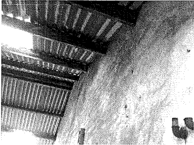
Photo 8. Detail of the dividing wall where the metal roof support beams adjoin
