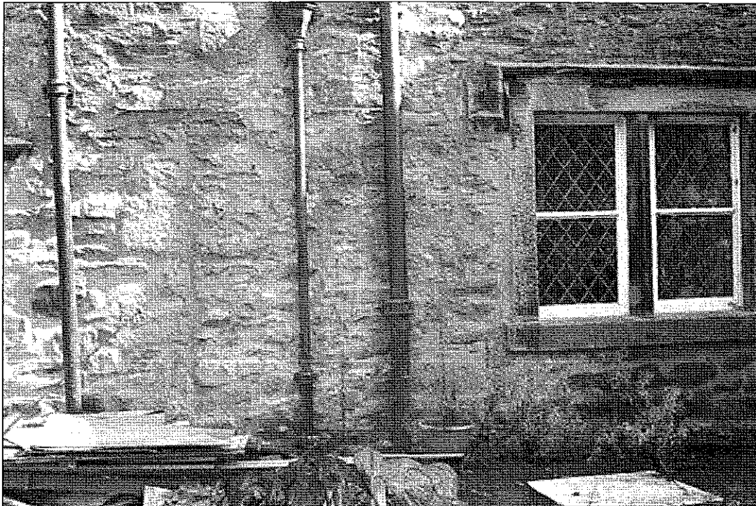
9 Evidence of blocked doorway to left of window
