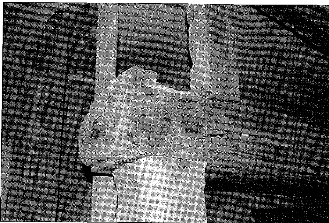
12. Detail of chamfered heck post supporting bressumer
