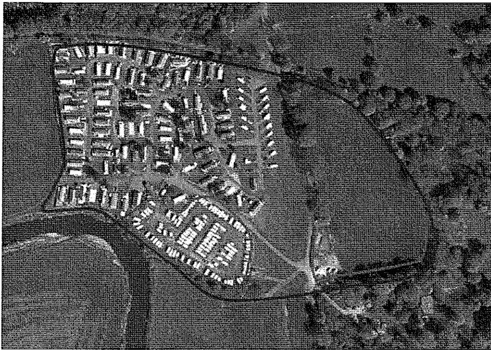
Figure 3: Aerial photograph showing site context of the caravan park
