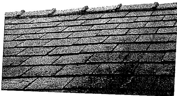
Roof is in general good order
