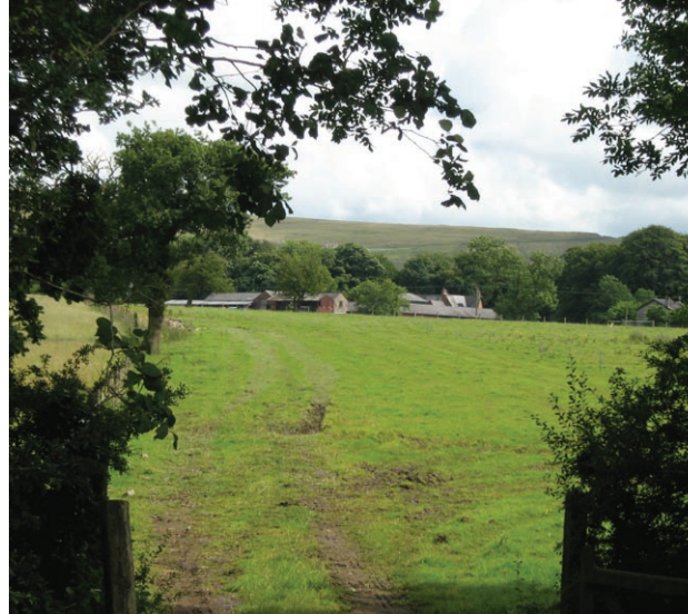
Higher Standen Farm Buildings
